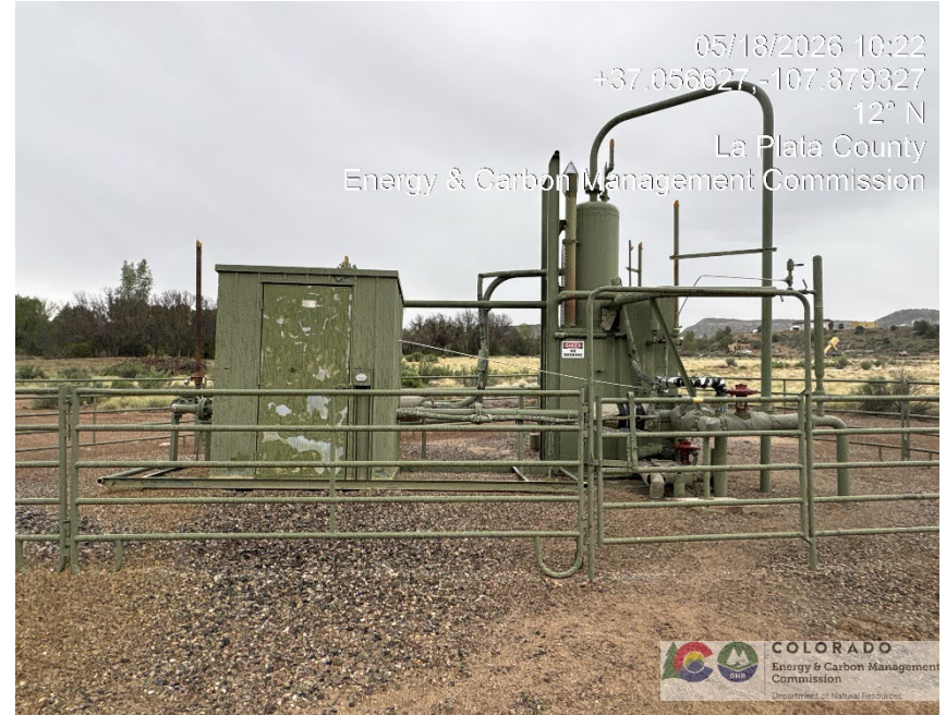
10. Meter run and vertical heated separator. Separator is anchored by turnbuckles connected to buried concrete and also by flow lines.
