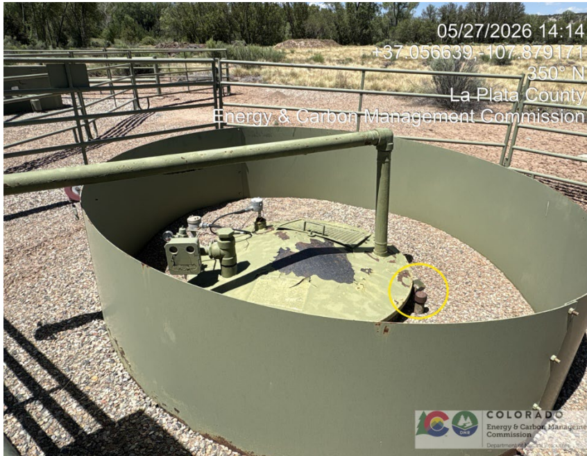
27. 21 BBL PBV tank in secondary containment showing single anchor tied down point observed. Paint on tank inadequate.
