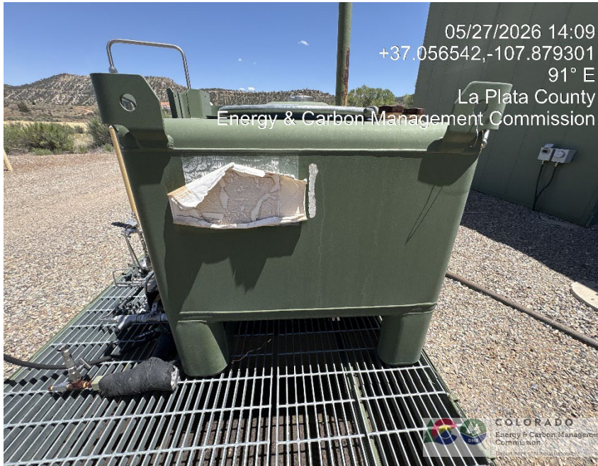
37. Chemical injection container. Manufacturer's label not legible. Contents unknown.
