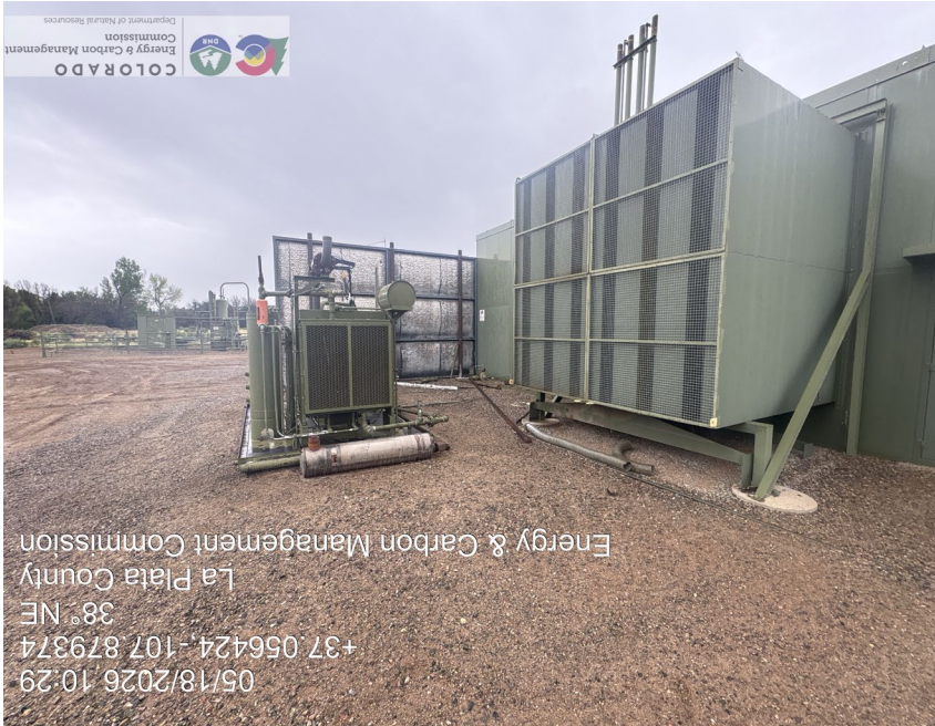
21. Skid mounted compressor (left) next to station structure lacks muffler and is noisy.
