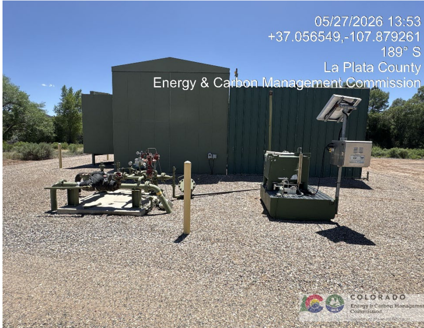
15. North side of compressor station looking south showing a midstream gas valve and regulator manifold on concrete pad and a chemical injection system on top of spill containment.
