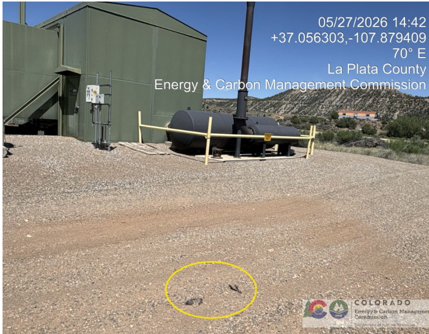
19. View of outside of compressor station. Liner debris observed.
