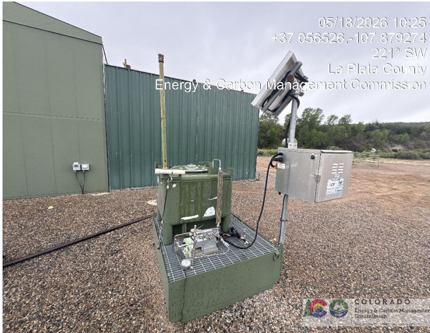
17. Chemical treatment container over spill prevention with solar telemetry on top of spill prevention. Manufacturer's labels not legible. Contents unknown. Est Vol ~50 gal.
