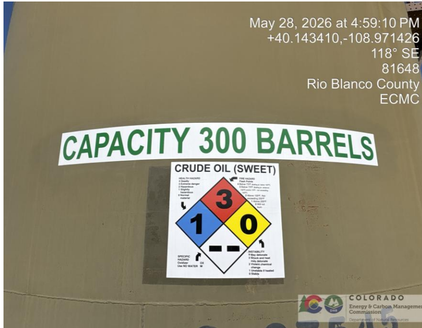
Photo # 5803 Production tank label lacks operator name & contact number
