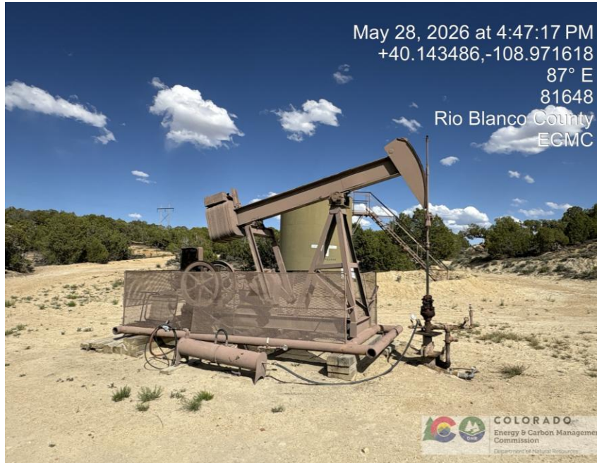
Photo # 5783 Weeds/undesirable plant species presents a potential fire hazard
