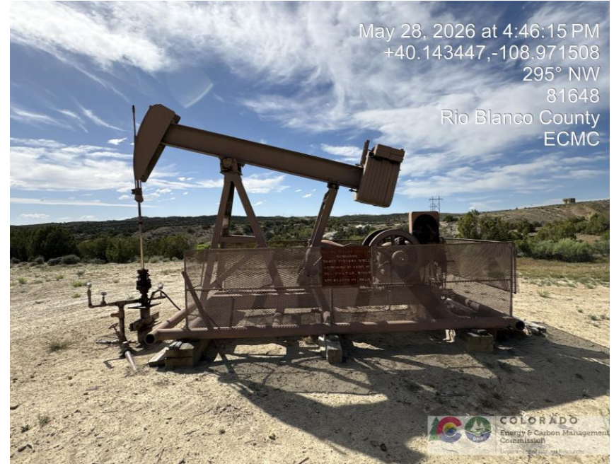
Photo # 5781 Weeds/undesirable plant species presents a potential fire hazard
