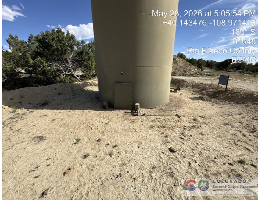
Photo # 5811 Weeds/undesirable plant species presents a potential fire hazard
