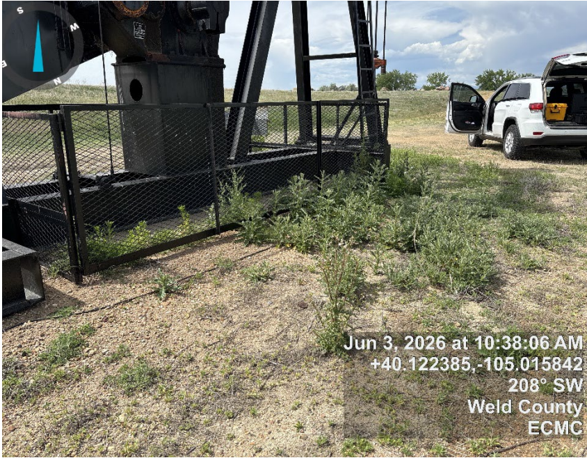
Photo 5: Overgrown, undesirable vegetation
