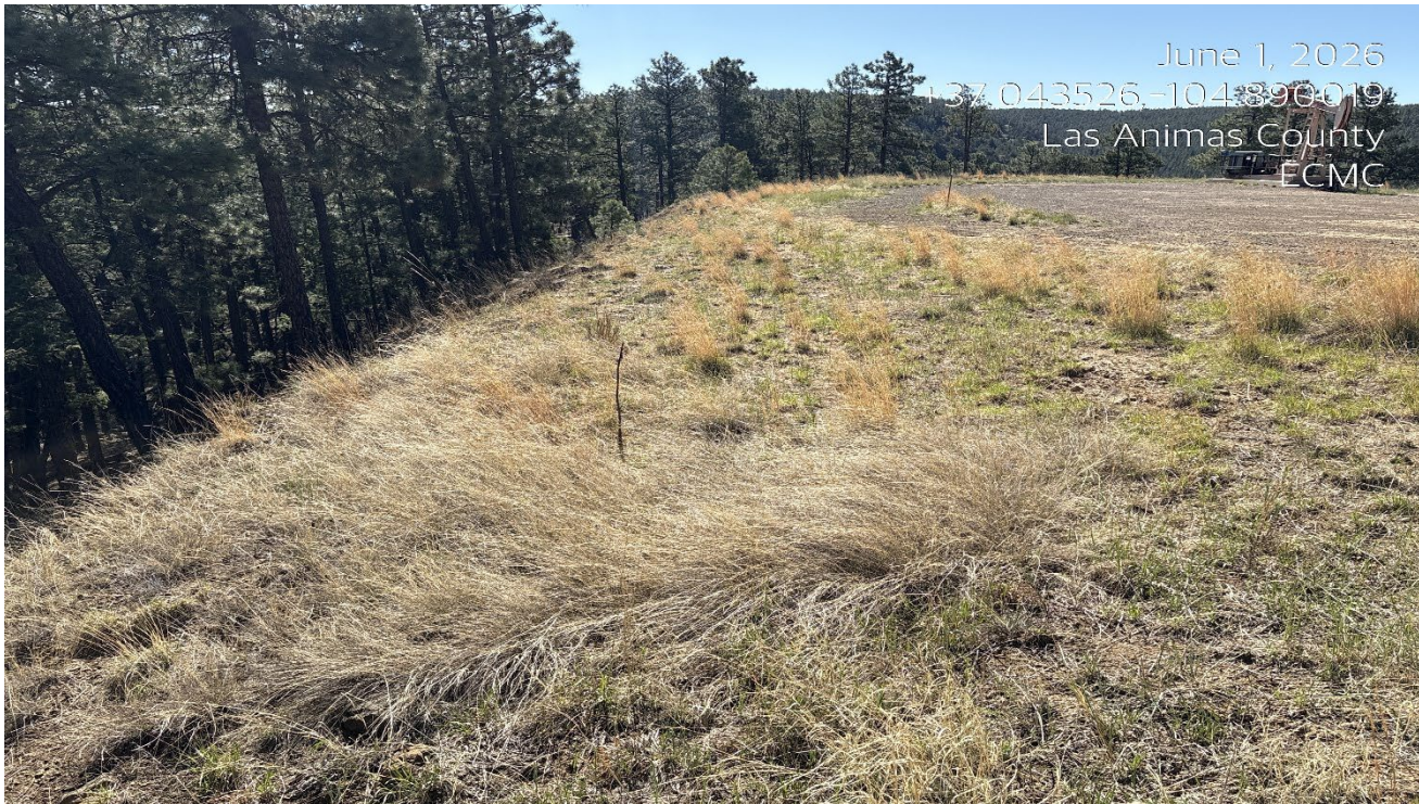
Photo 2. Facing east along the fil slope which is stabilized with vegetation.
