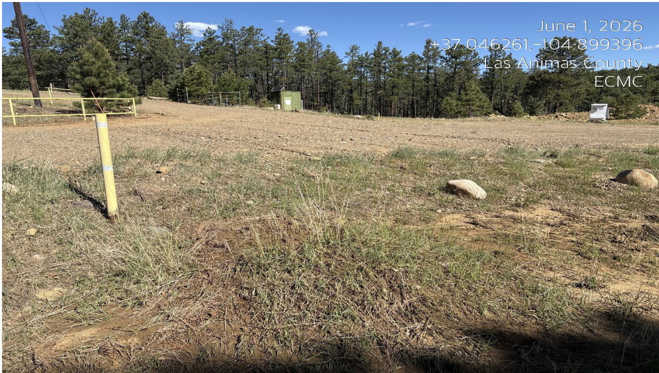
Photo 2. This culvert outlet is filled in and needs maintenance.
