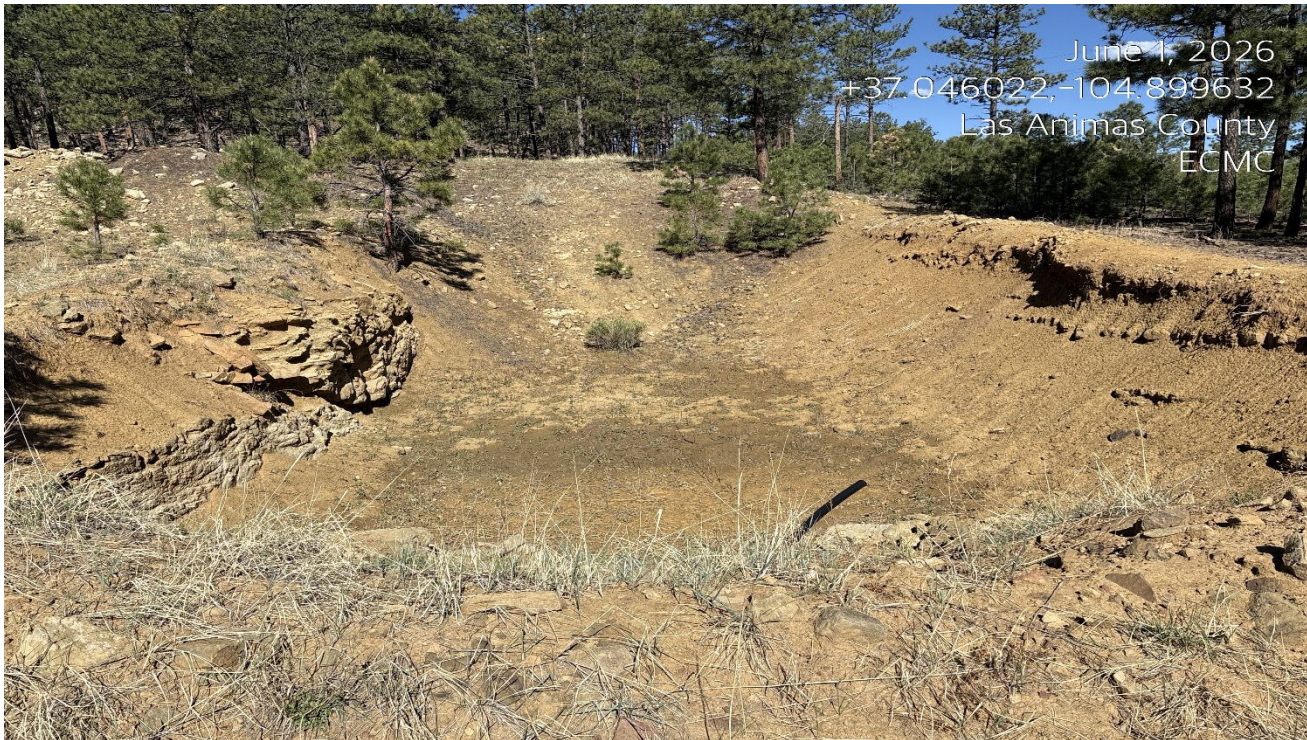
Photo 2. Facing west. The associated pit of the Hill Ranch 33-4 has not been backfilled and reclaimed.
