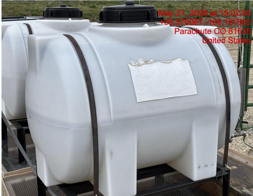
Weathered/Illegible Labeling on Chemical Tank – Photo #03976
