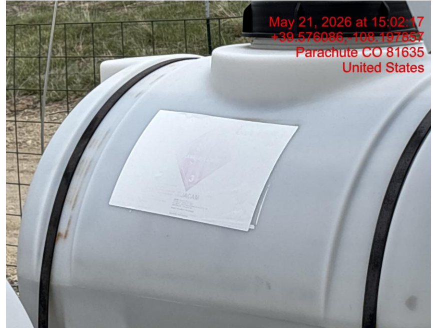
Weathered/Illegible Labeling on Chemical Tank – Photo #03977
