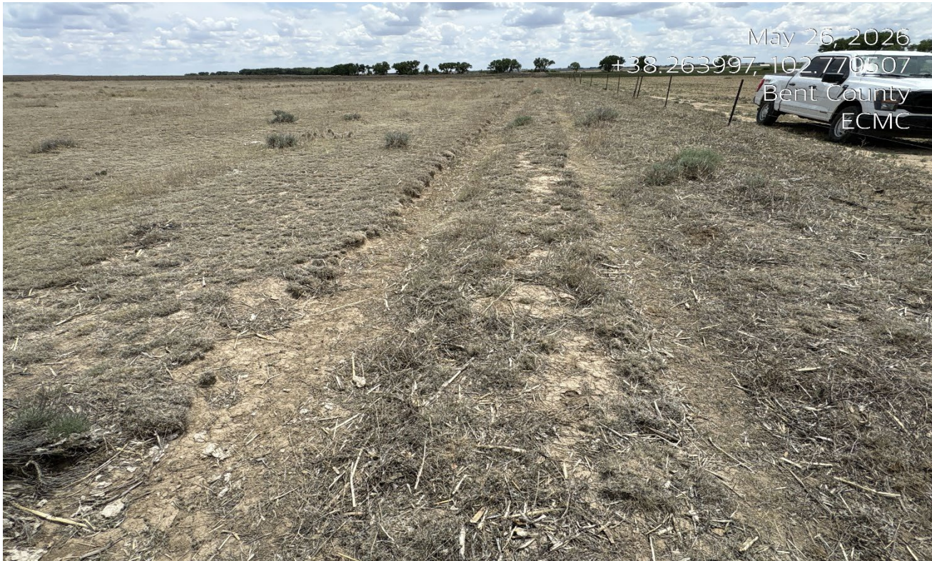
Photo 2. Facing north along the two track road. The vehicle ruts need to be filled in with soil for proper contouring.
