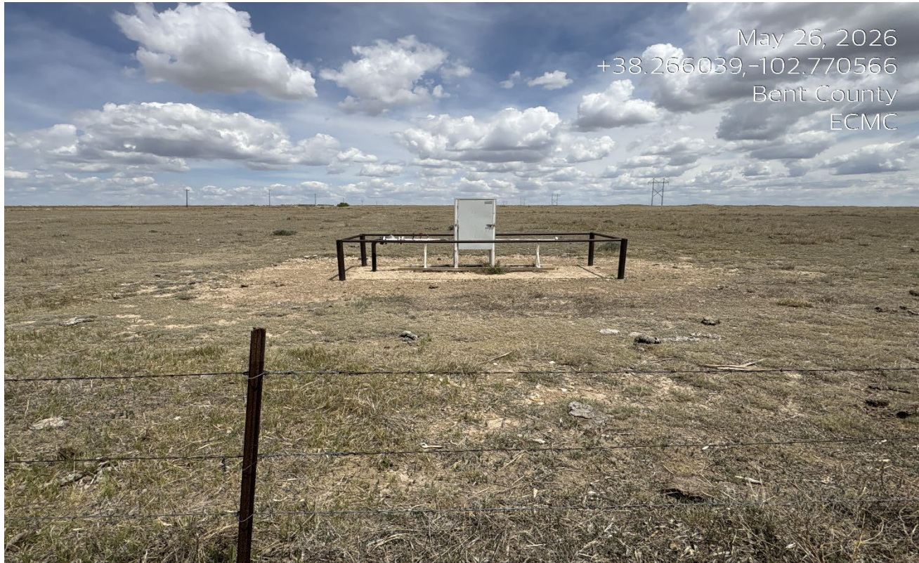
Photo 1. The meter flowline riser located along the access road has not been removed.
