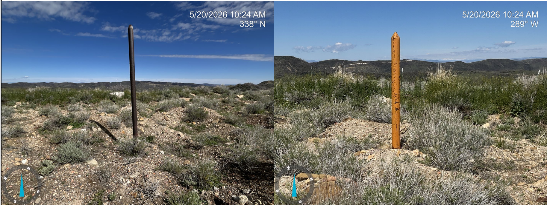
Photo 3: Photos showing the plugged & abandoned well markers at the location.
