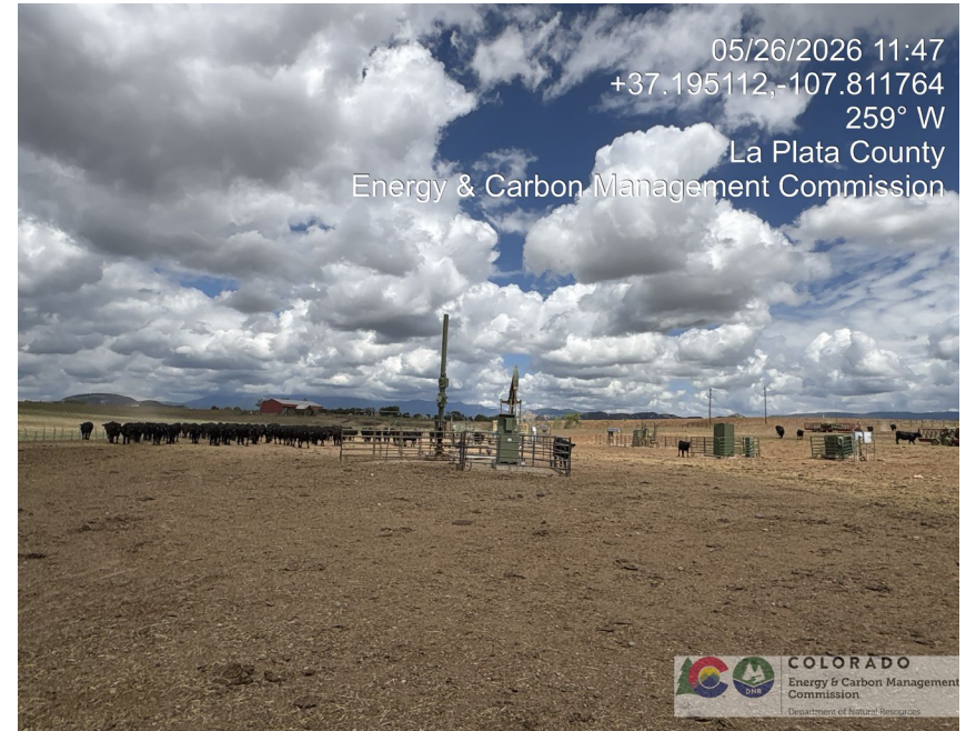
28. Well site overview from southeast corner looking west.
