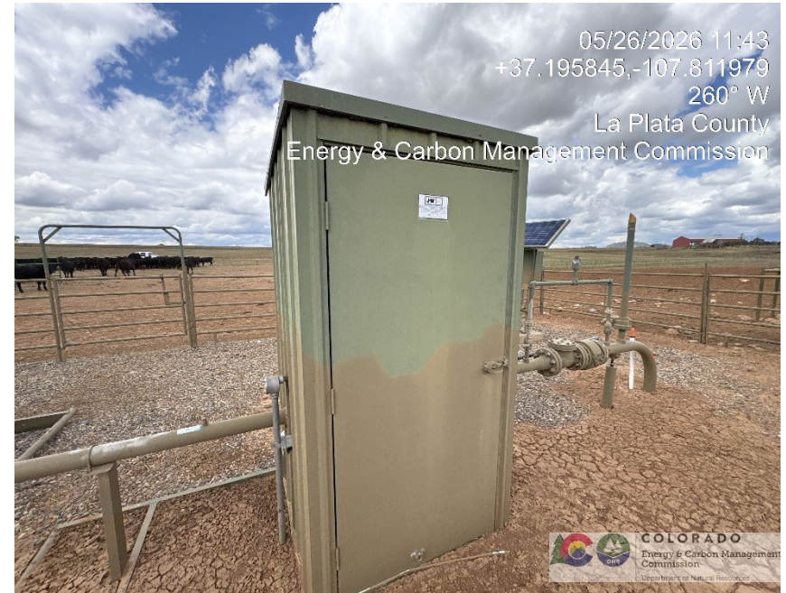
22. A4 meter shed.
