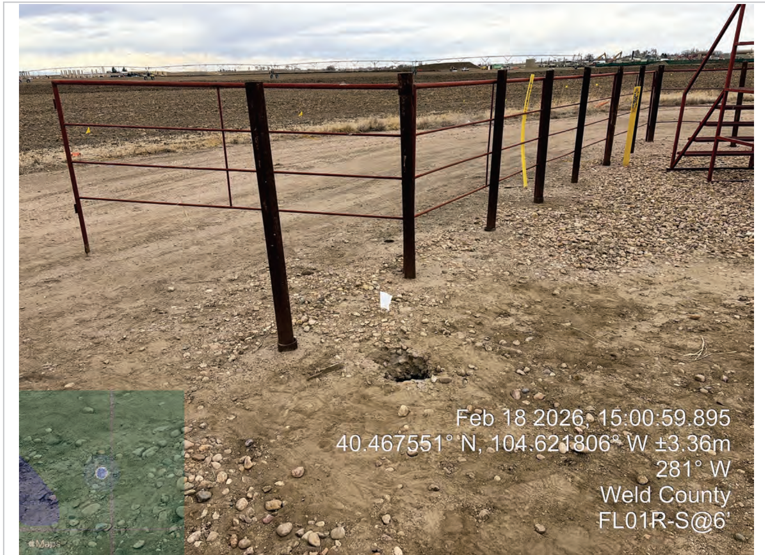
FL01R-S: View West
