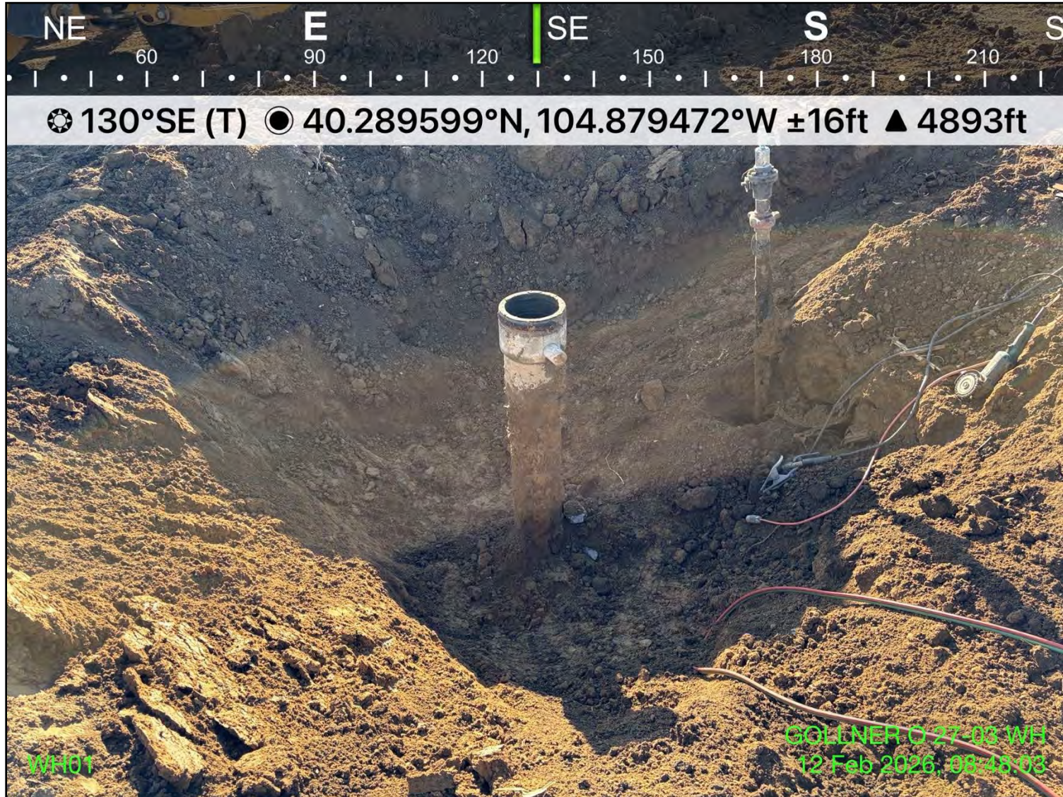
Photo 2: View of wellhead excavation extent, facing southeast
