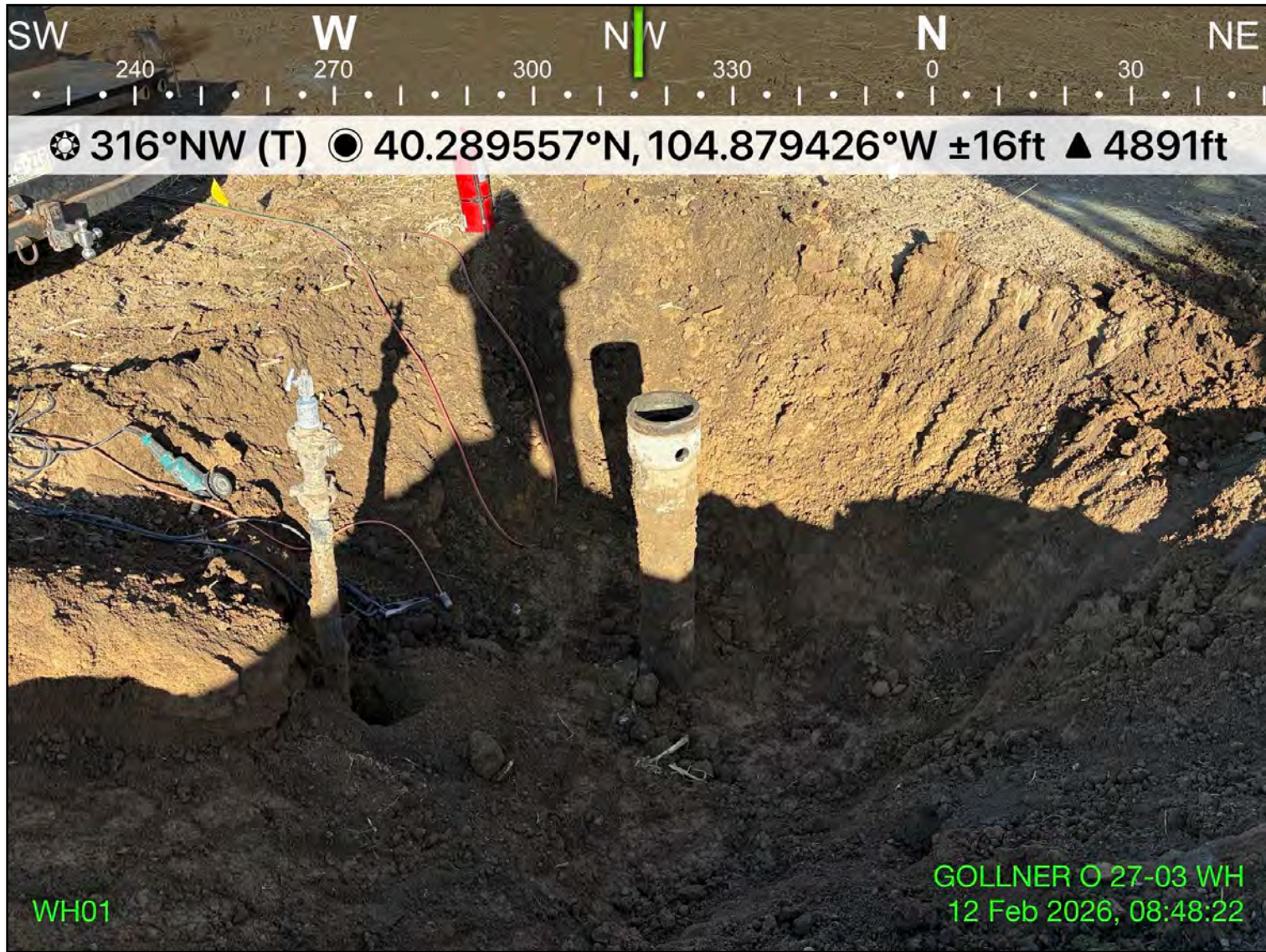
Photo 4: View of wellhead excavation extent, facing northwest
