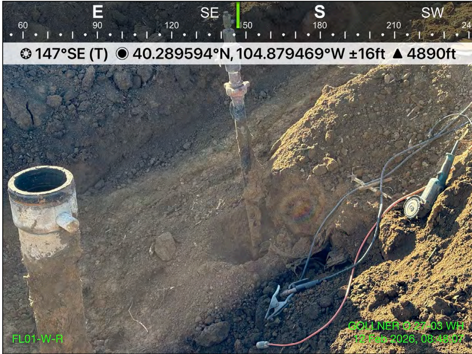
Photo 5: View of FL01-W-R sample location inside wellhead excavation extent, facing southeast
