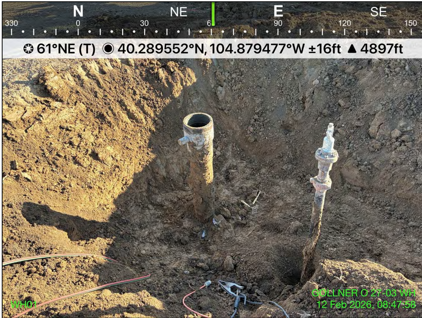
Photo 1: View of wellhead excavation extent, facing east-northeast
