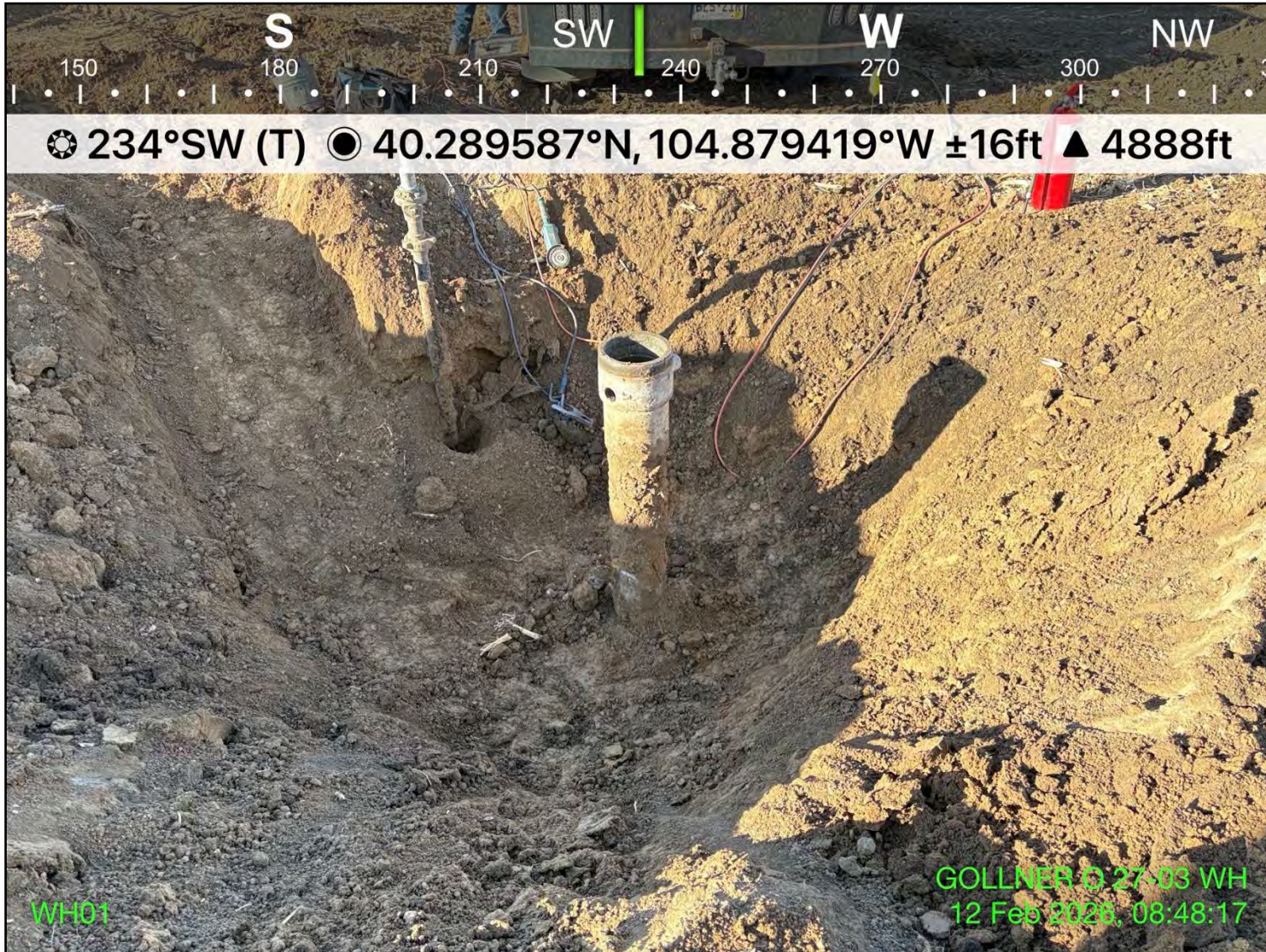
Photo 3: View of wellhead excavation extent, facing southwest
