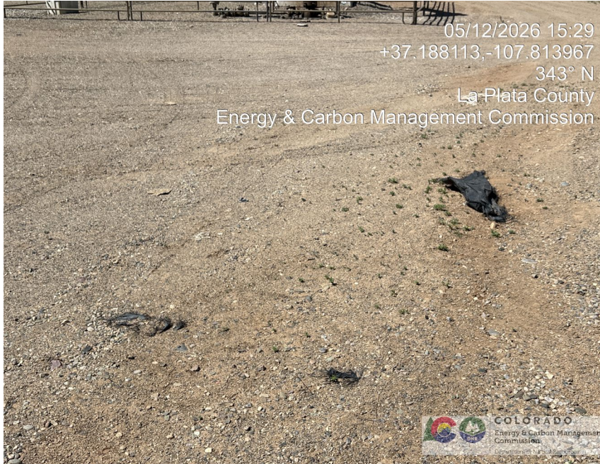
23. One of many examples of liner material observed.
