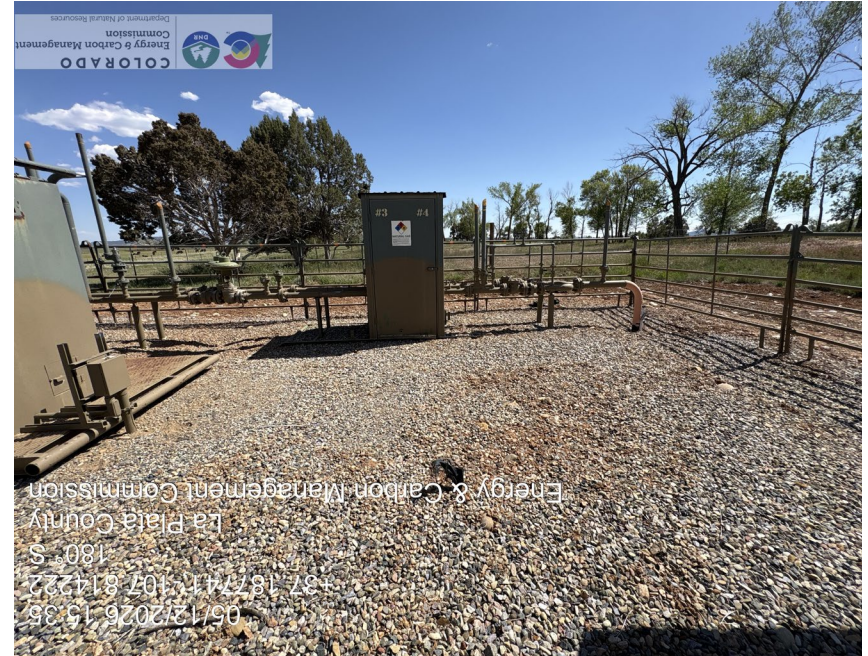
24. Another example of liner material observed.
