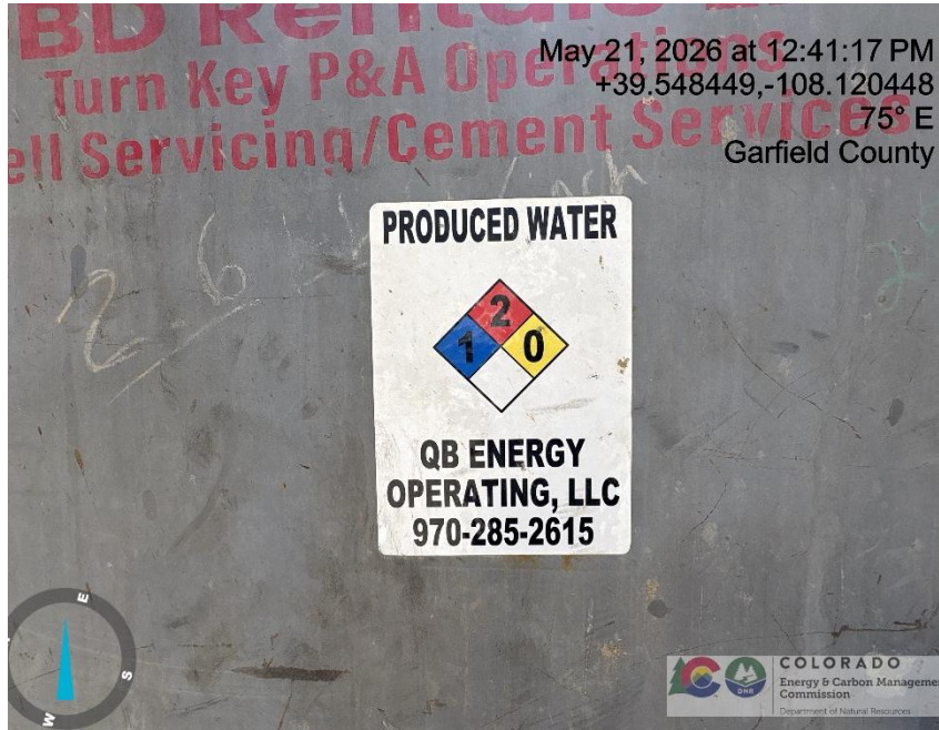
Photo # 1293 Label on rig tank lacks capacity
