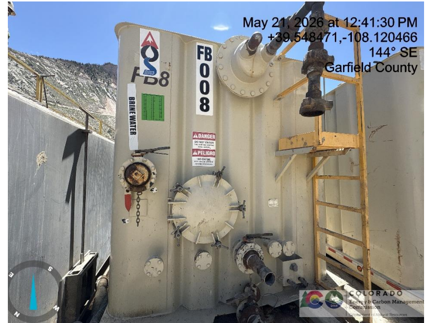
Photo # 1294 Frac tank lacks required labeling
