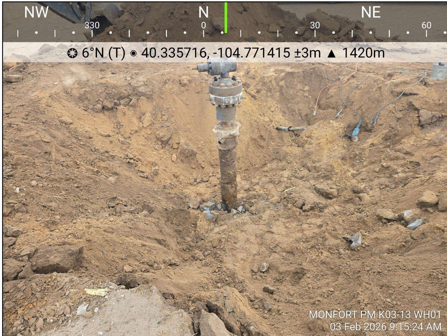
Photo 3: View of excavation, facing north
