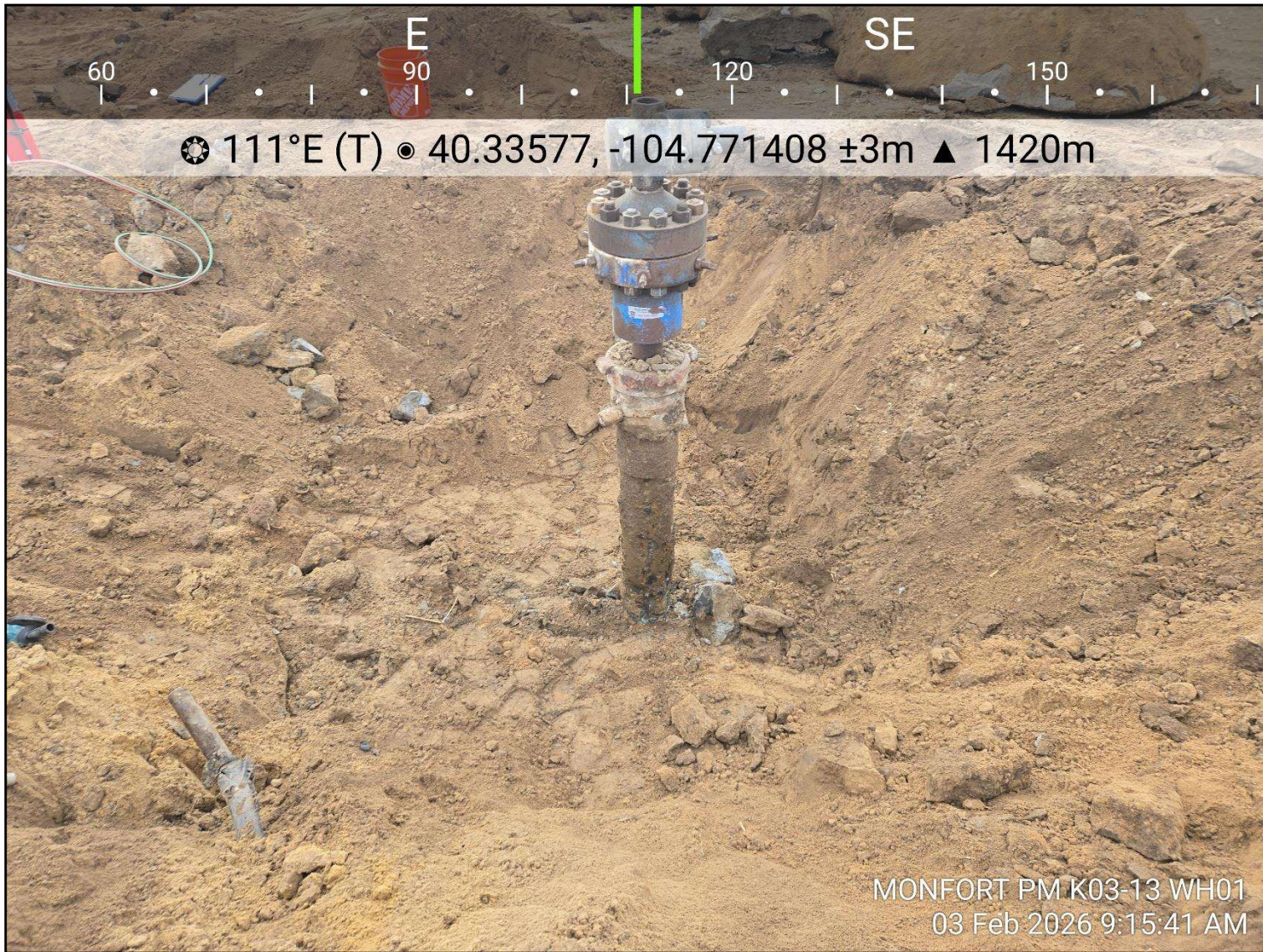
Photo 1: View of excavation, facing east-southeast
