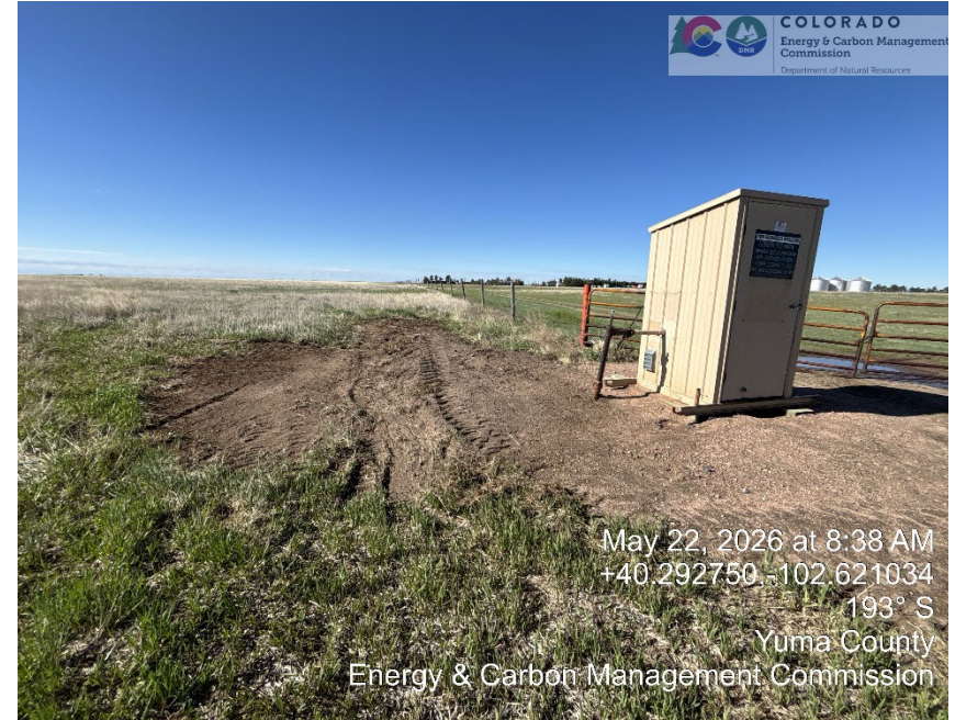
Meter shed removed
