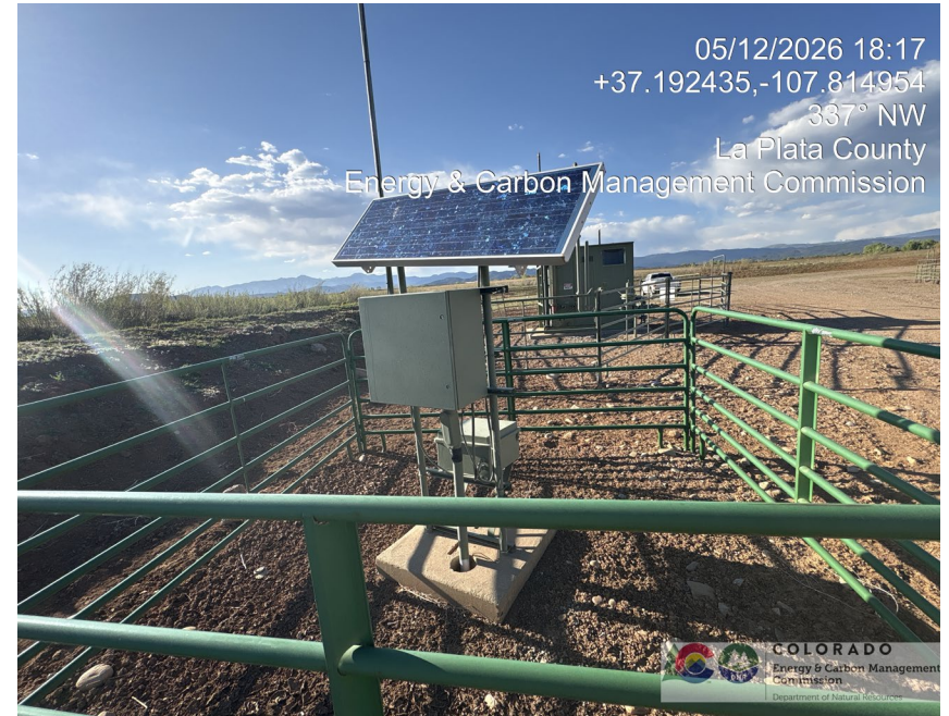
10. Solar telemetry for production equipment.
