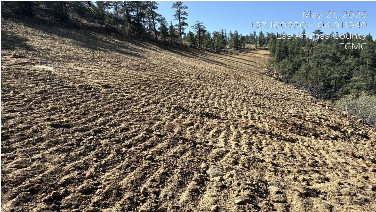
Photo 2. Facing south further along the reclamation area. The soils have been tracked seeded, and mulched.
