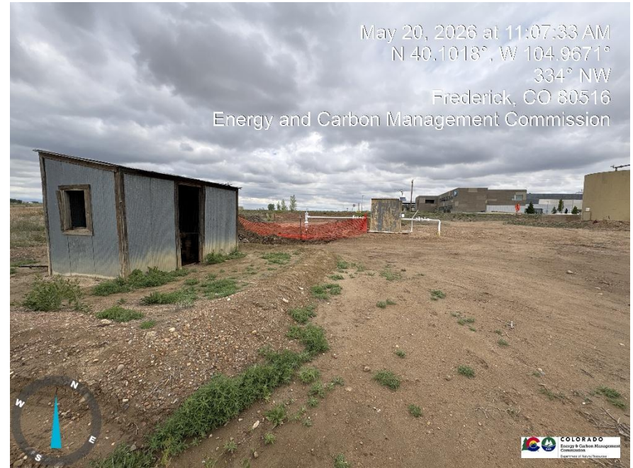
View from location looking north toward fenced excavation at the Western Midstream gas meter run. The KPK outbuilding houses a flowline manifold.
