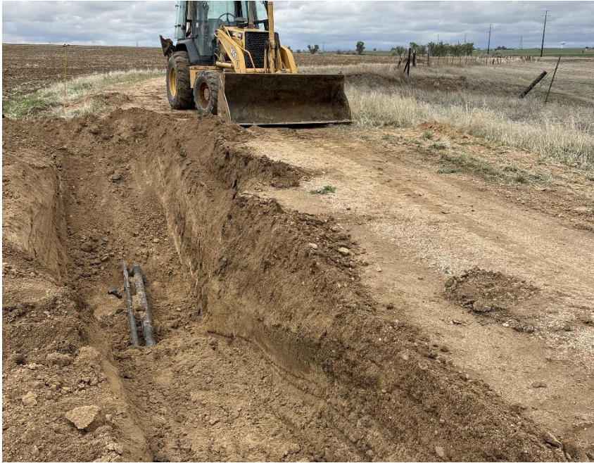
Eastern bell hole excavation exposing (1) 4" CS and (1) 2" CS off location flowlines approximately 350' east of spill/ release point @ 40.07180, -104.8940.
