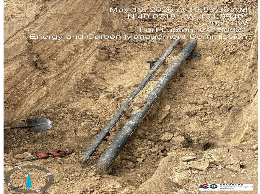
Closer view of (2) flowlines exposed in excavation
