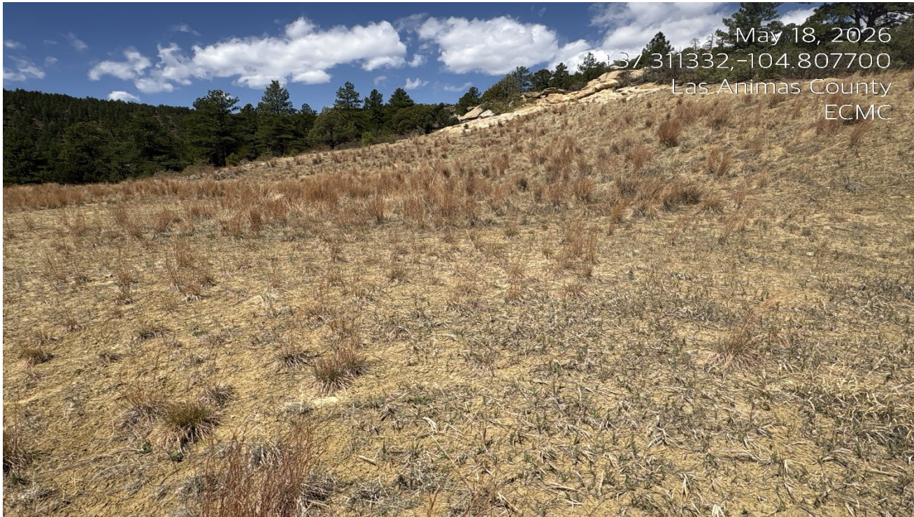
Photo 7. Facing northwest toward the fill slope which is stabilized with desirable vegetation.
