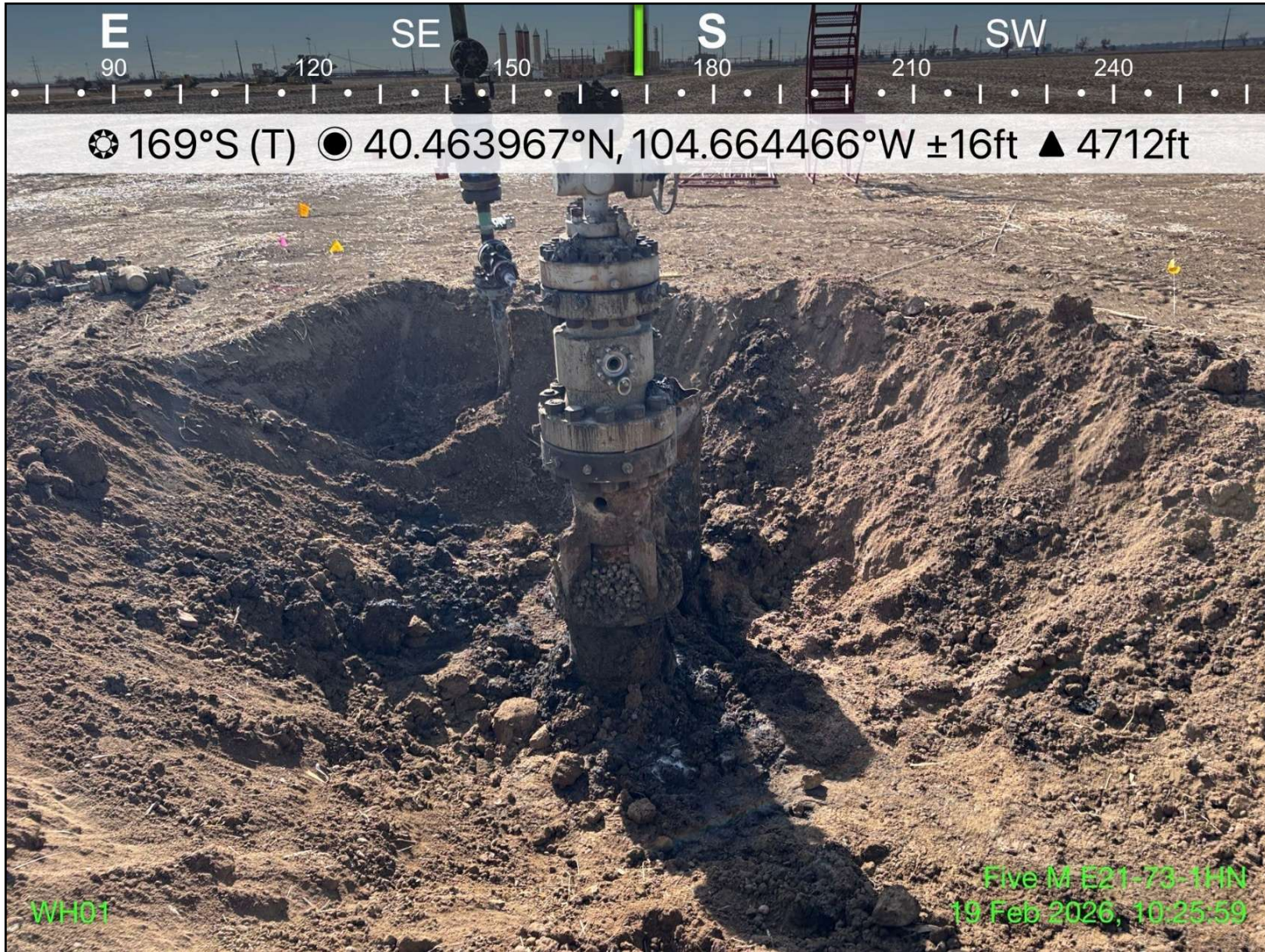
Photo 1: View of wellhead excavation extent, facing south
