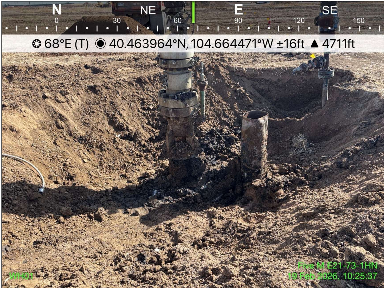
Photo 4: View of wellhead excavation extent, facing east-northeast
