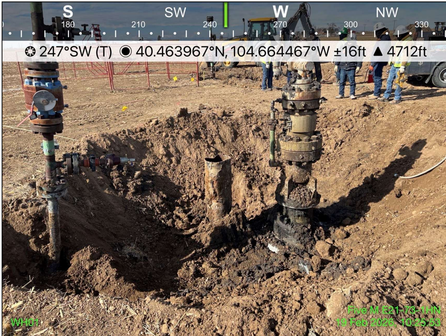
Photo 2: View of wellhead excavation extent, facing west-southwest
