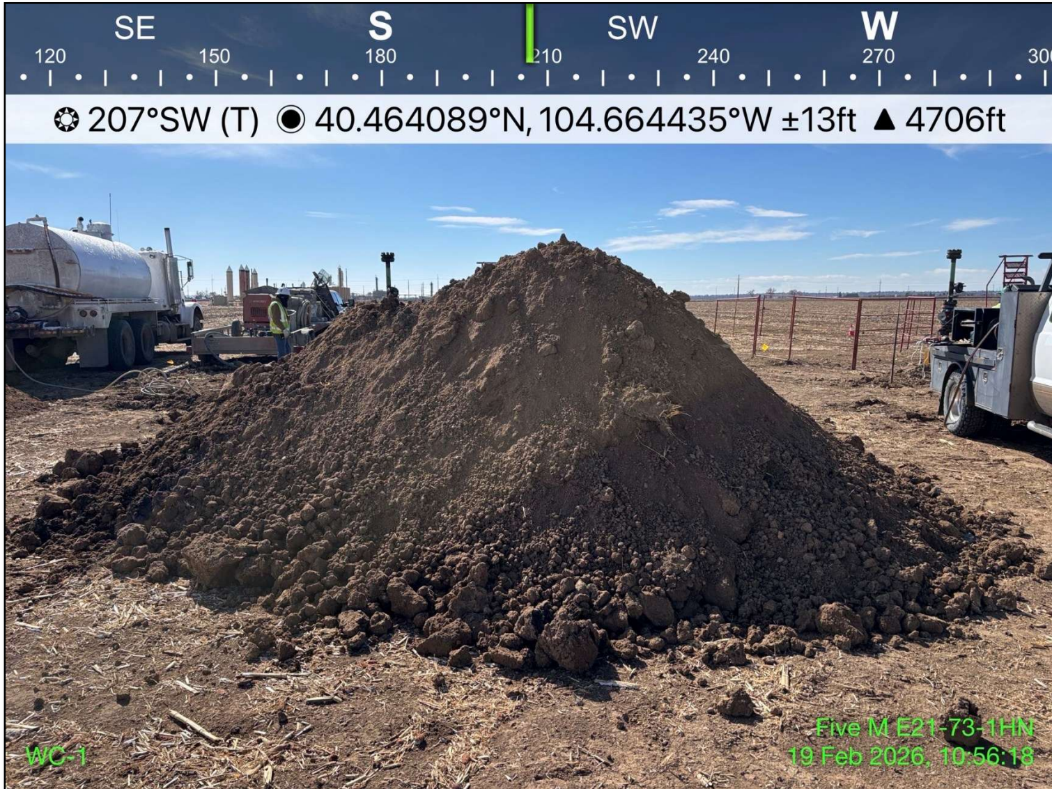
Photo 6: View of excavated soils stockpile and WC-1 sample location, facing south-southwest
