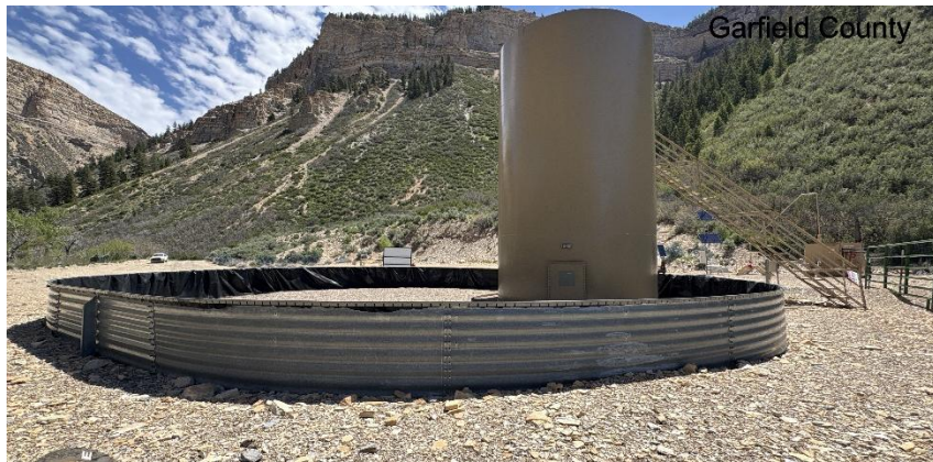
South West corner of location.
