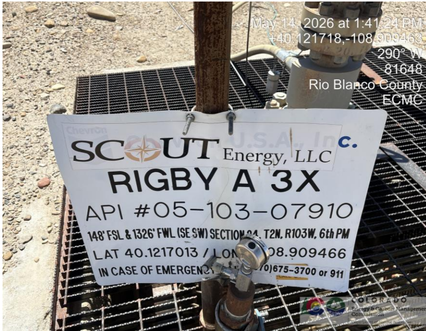
Photo # 5220 Wellhead sign lacks public road used to access the well
