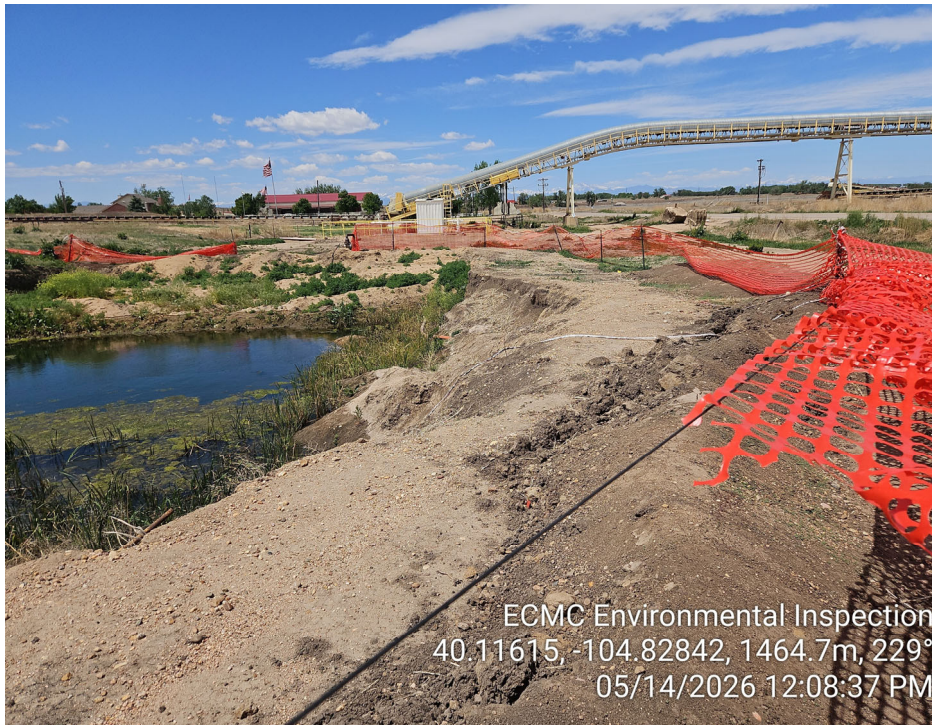
Photo 5 – Fencing down/inadequate around open excavation.
