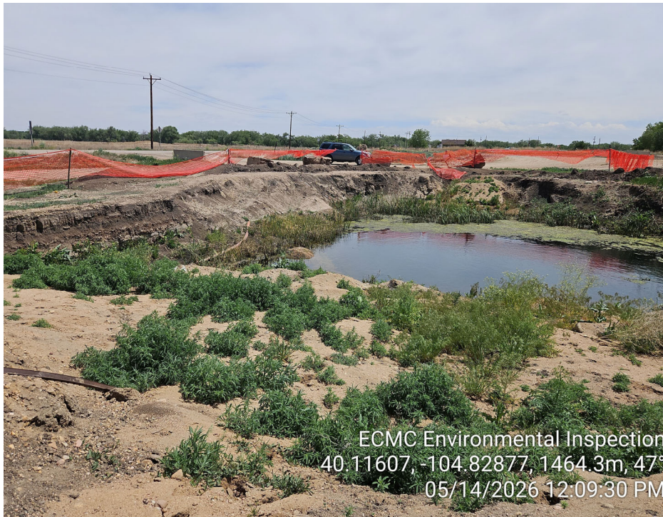
Photo 9 – Open excavation. Groundwater/weeds present in open excavation. Fencing down/inadequate. Portions of old flowline visible on open excavation (trash).
