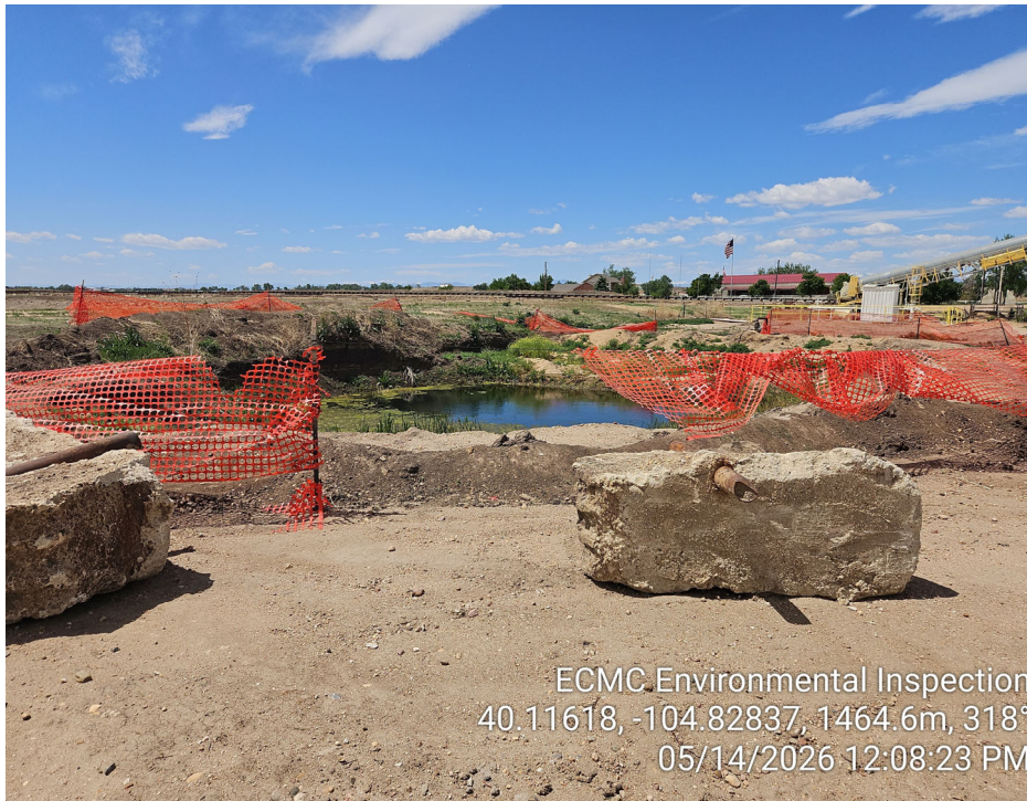
Photo 3 – Open excavation. Downed/inadequate fencing.
