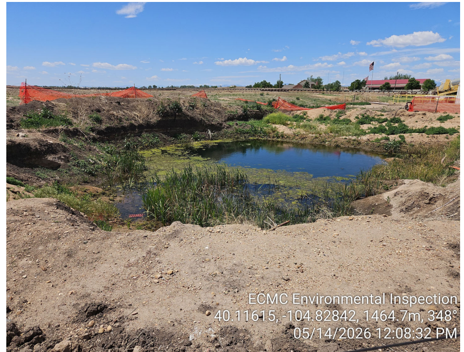
Photo 4 – Open excavation. Groundwater/weeds present in open excavation. Fencing down/inadequate.
