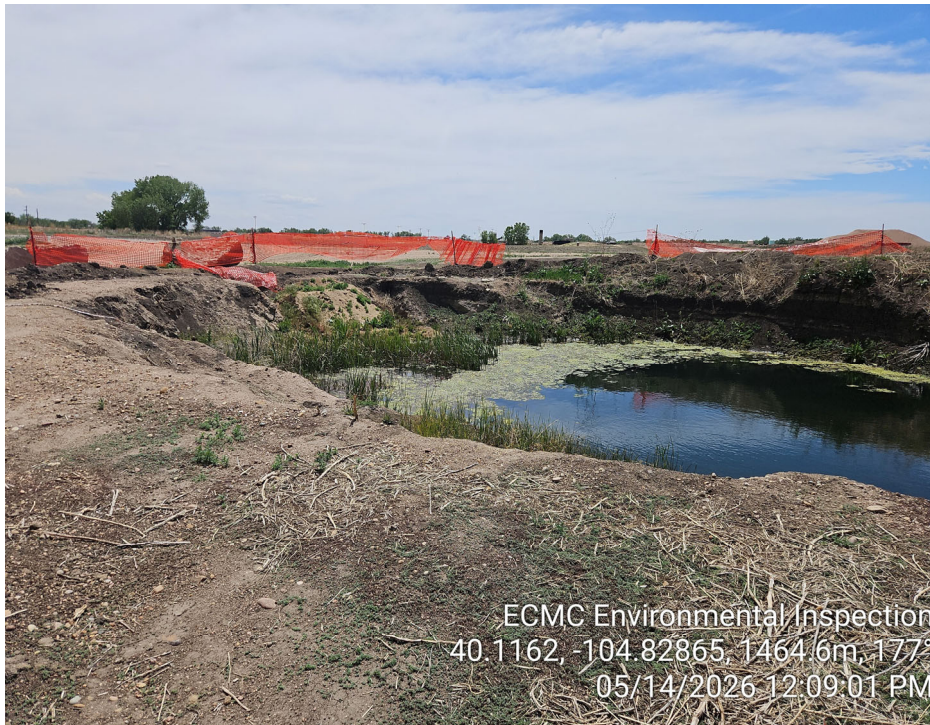
Photo 7 – Open excavation. Groundwater/weeds present in open excavation. Fencing down/inadequate.
