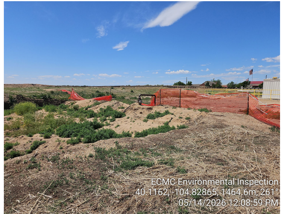
Photo 6 – Fencing down/inadequate around open excavation.
