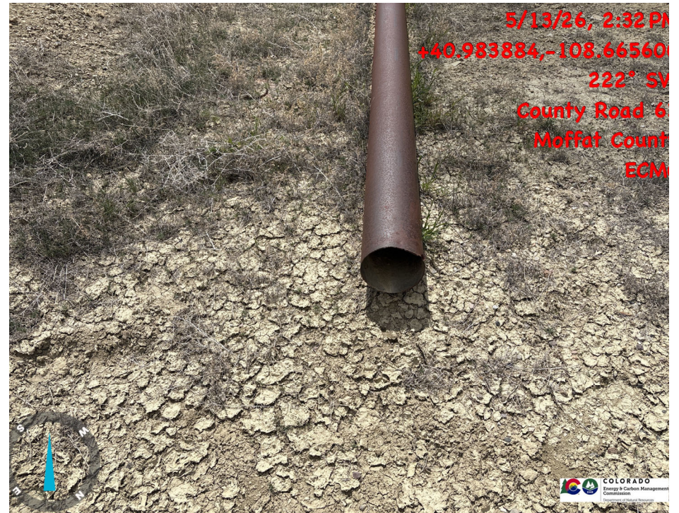
Debris has open ended for wildlife to enter
