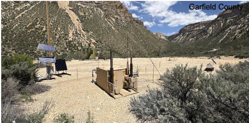
South West corner of location.
