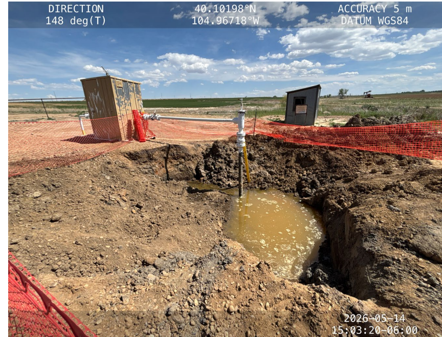
Excavation near the Meter House. Groundwater within excavation
