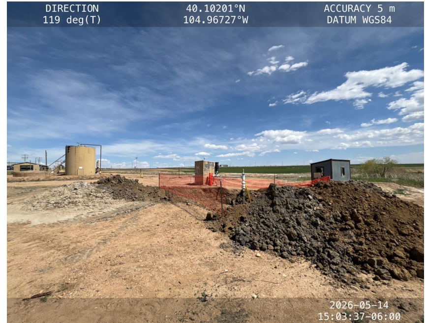
Excavation near the Meter House
