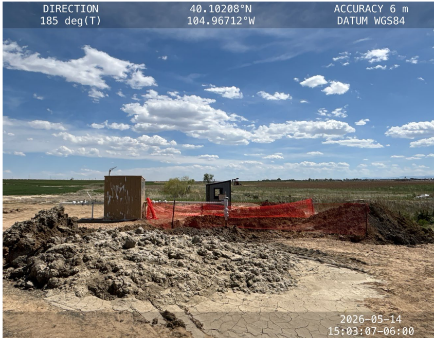
Excavation near the Meter House
