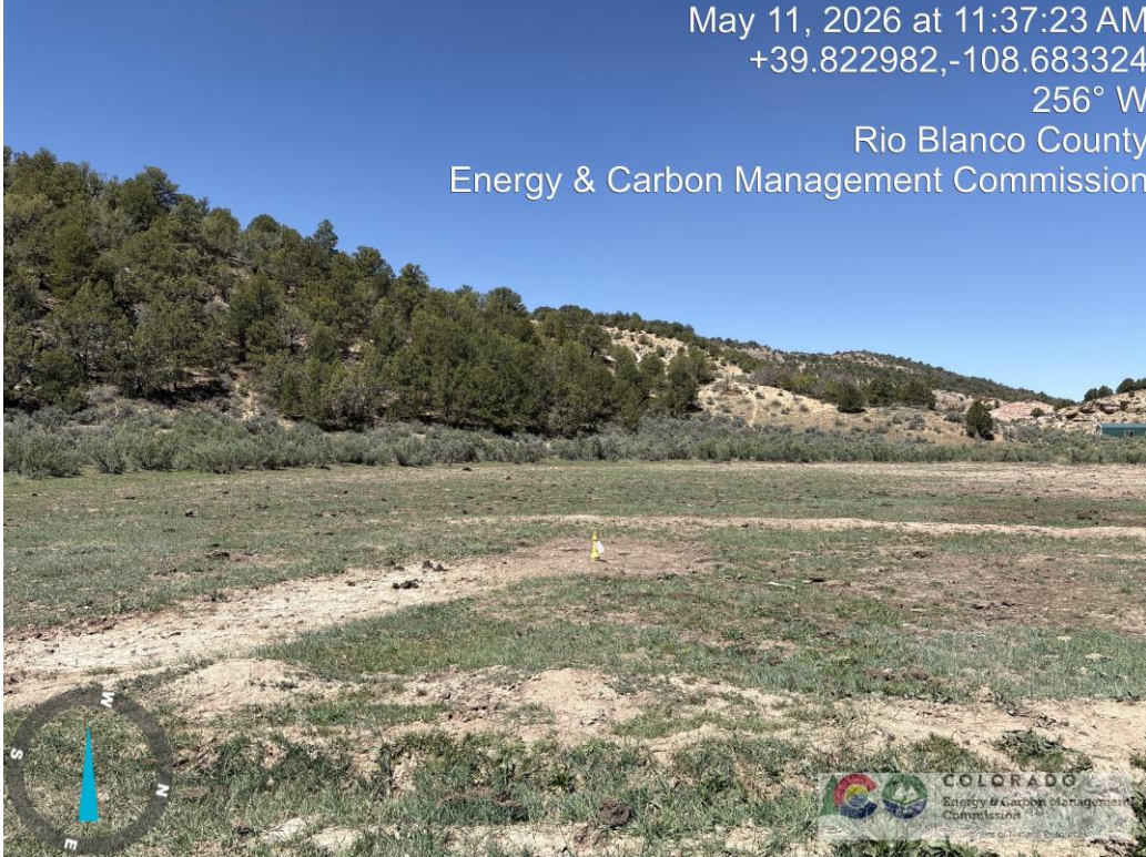
OOSLAT on pipe riser painted bright color.
