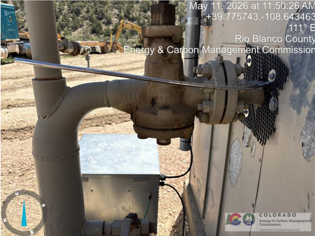
Oily residue on valve.
