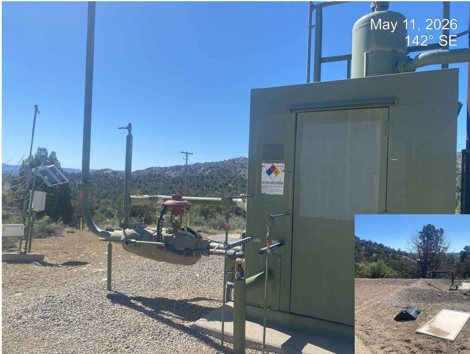
Photo 3. Label is starting to deteriorate, produced water sign has fallen off stand.
