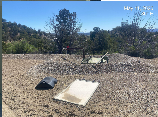
Photo 3. Label is starting to deteriorate, produced water sign has fallen off stand.
