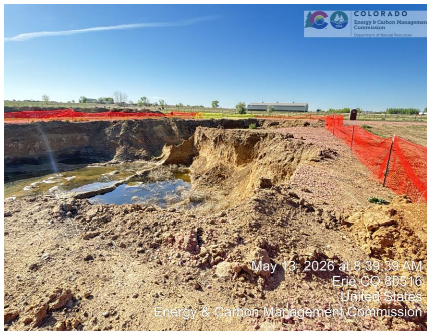
Photo 1 facility remediation at UPRR B 7 site
