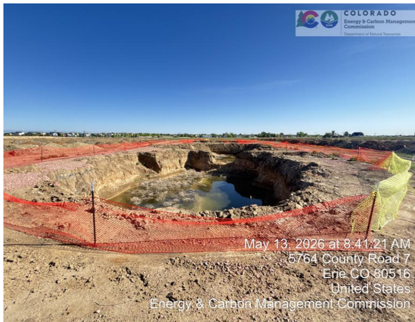
Photo 3 facility remediation at UPRR B 7 site
