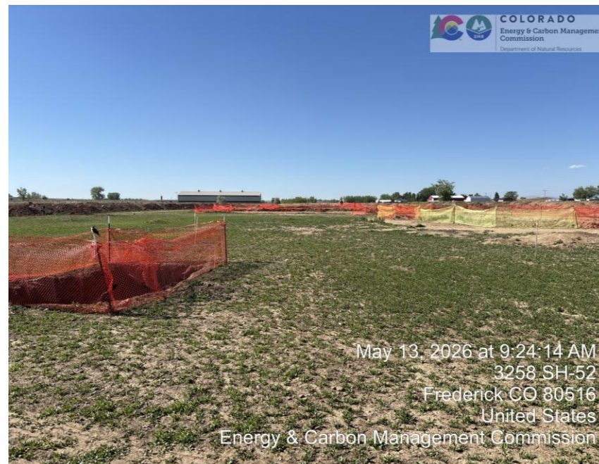
Photo 4 facility remediation at UPRR B 7 site
