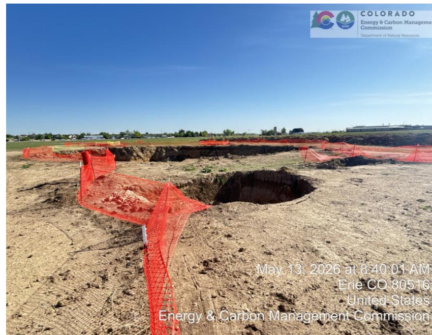
Photo 2 facility remediation at UPRR B 7 site
