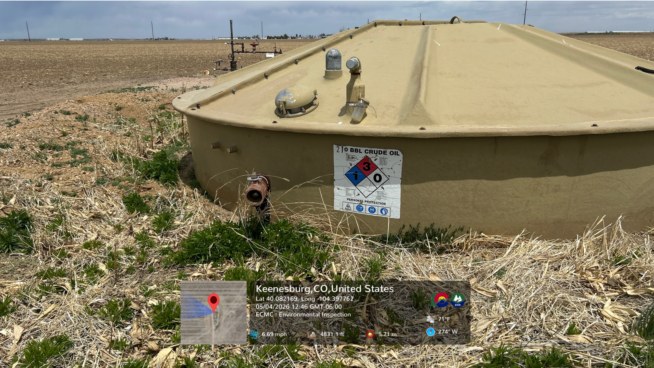
The partially buried fiberglass tank is labeled as 210 bbl crude oil.
