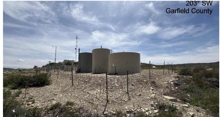
North East corner of location.
