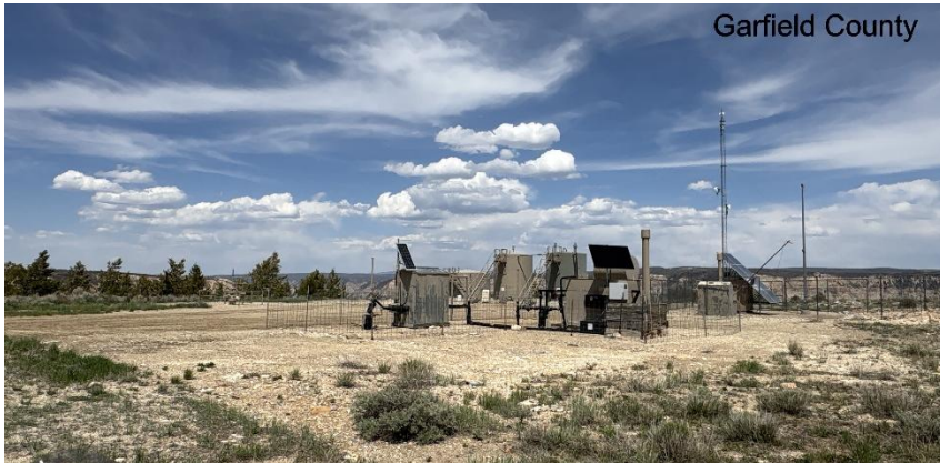
South West corner of location.
