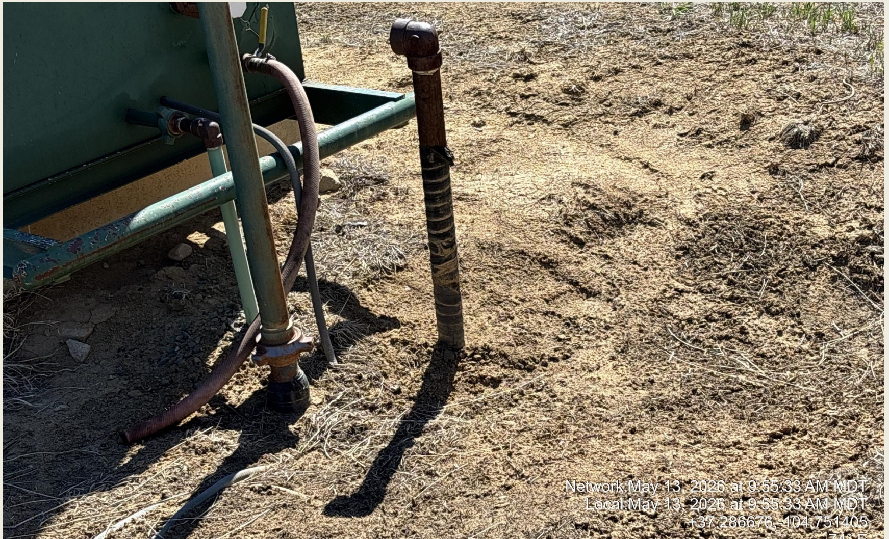
PHOTO 6: UNUSED EQUIPMENT (2" RISER NEAR METER HOUSE NOT LABELED). REMOVE OR LABEL RISERS PER RULE 606. CA DATE 6/13/2026.
