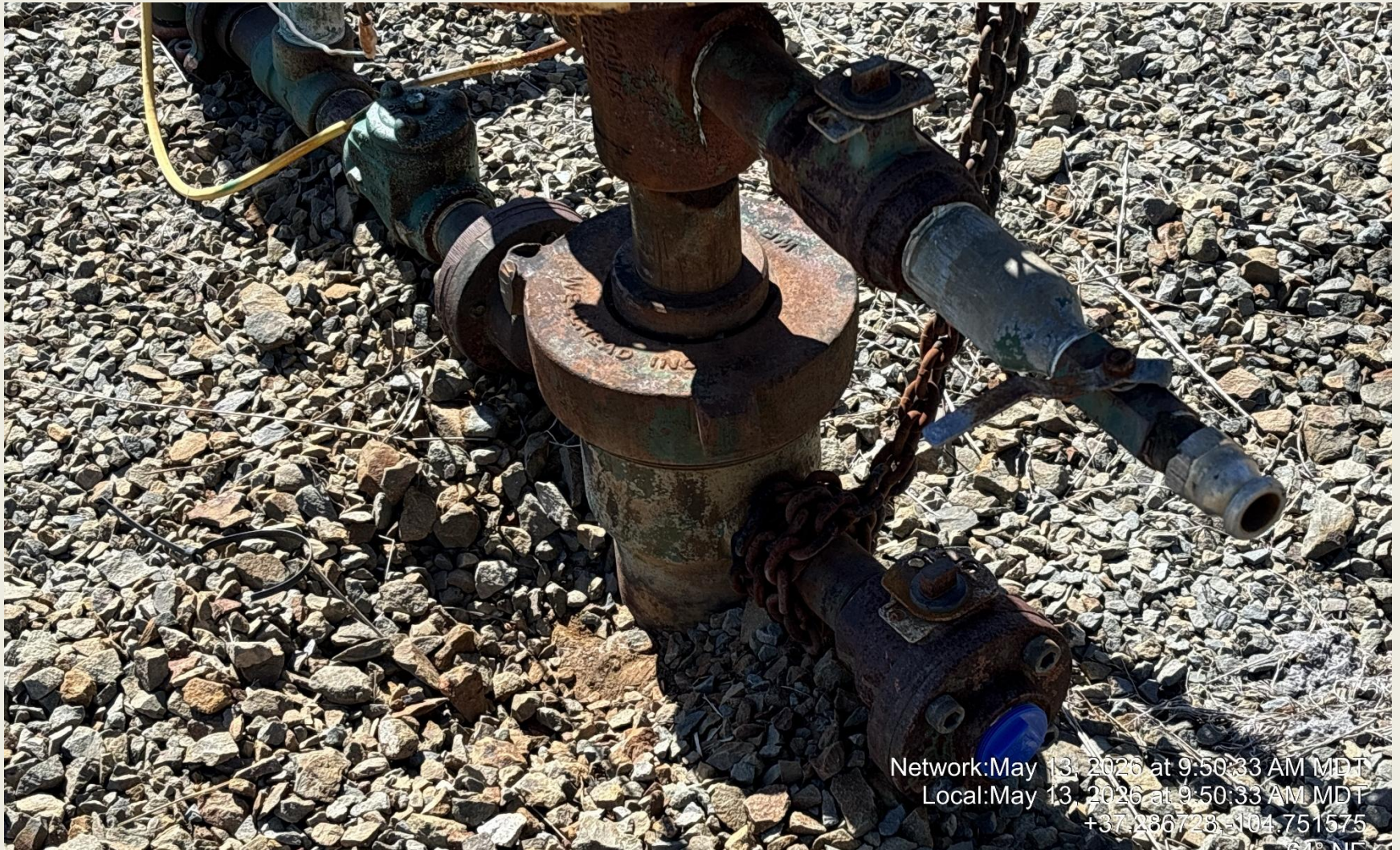
PHOTO 13: Bradenhead inaccessible or not visible. Install appropriate fittings to allow bradenhead visual inspection as per Rule 419.a.(1), (2). ALL WELLS SHOULD HAVE ACCESS TO BRHD BY NOW CA DATE 5/15/2026.
