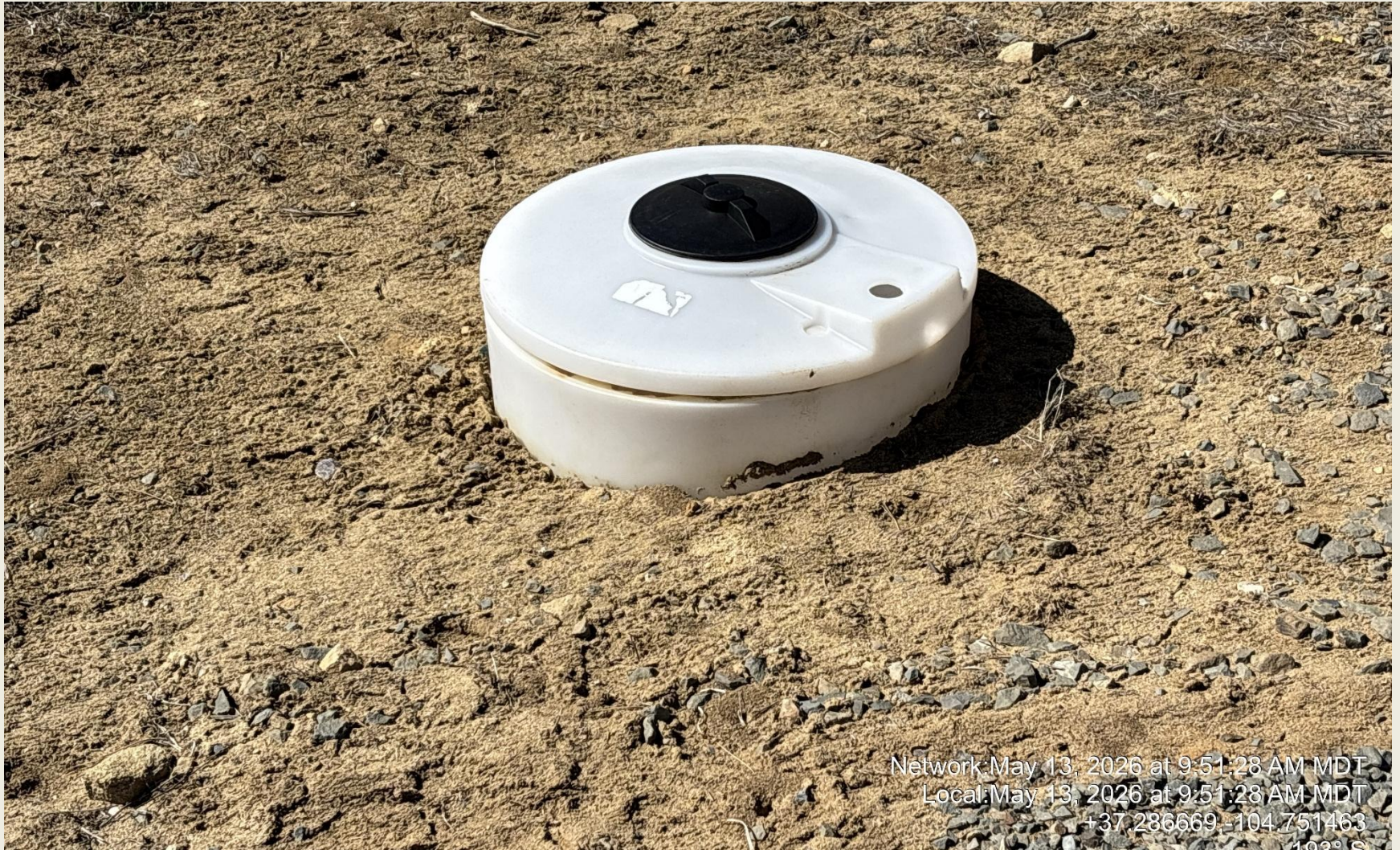
PHOTO 8: UNUSED EQUIPMENT (IN GROUND DRIP TANK NO LONGER IN USE). REMOVE UNUSED EQUIPMENT PER RULE 606. CA DATE 6/13/2026.
