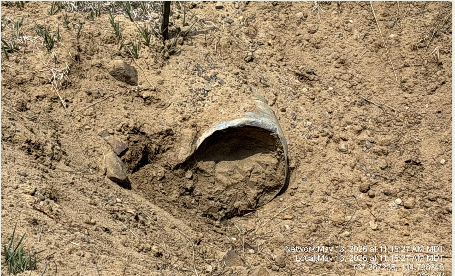
PHOTO 10: CULVER AT ENTRANCE OF LOCATION IS PLUGGED. CLEAN CULVER PER RULE 1002. CA DATE 6/13/2026.
