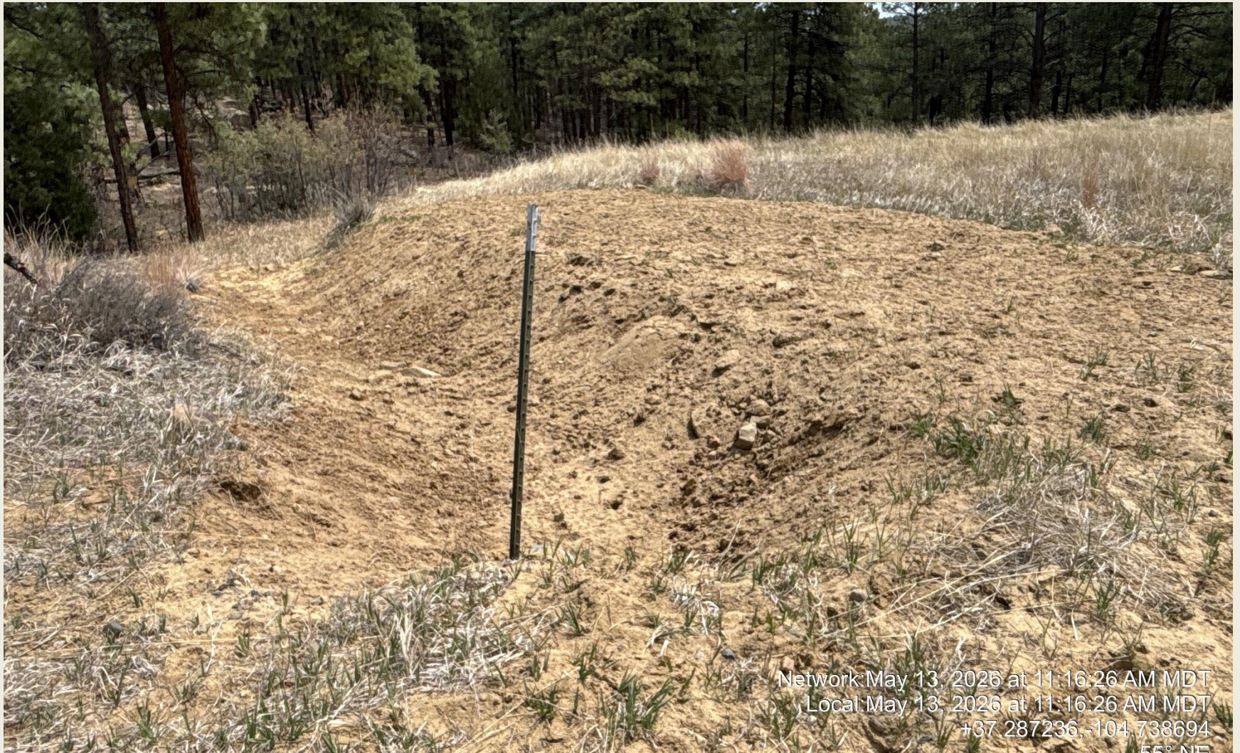
PHOTO 11: RECENT RECLIMATION AREA DISTURBANCE DOES NOT APPEAR TO HAVE BEEN RESEEDED. SEED DISTURBED AREA PER RULE 1003. CA DATE 7/15/2026.
