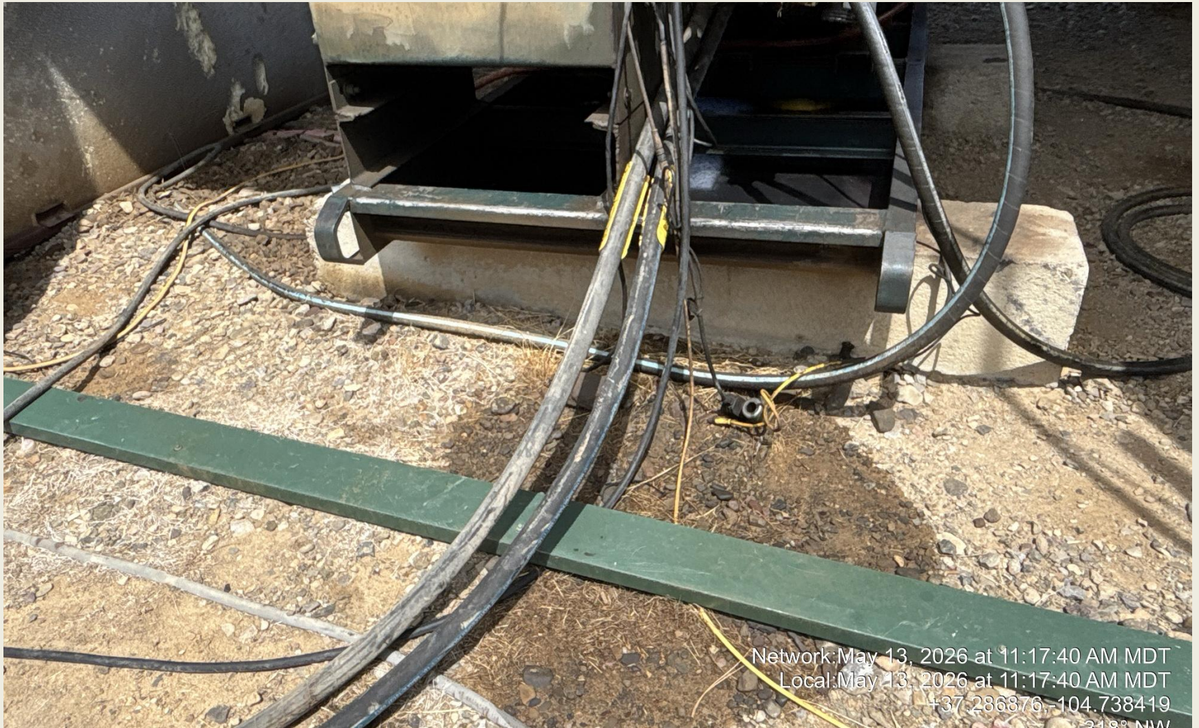
PHOTO 7: AREA OF IMPACTED SOIL NEAR PRIME MOVER SKID. AT TIME OF INSPECTION THIS EQUIPMENT IS NOT IN OPERATION HOWEVER IT APPEARS TO HAVE SIGNIFICANT OIL LEAKS THAT SHOULD BE REPAIR PRIOR TO PUTTING EQUIPMENT BACK IN USE. Conduct maintenance on equipment, cleanup stained material and review self inspection processes. COMPLY WITH RULE 1002,.(2).D CA DATE 6/13/2026.
