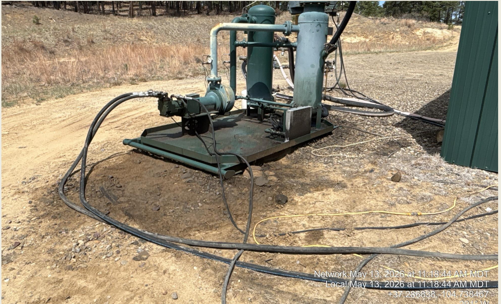
PHOTO 8: AREA OF IMPACTED SOIL NEAR COMPRESSOR SKID. AT TIME OF INSPECTION THIS EQUIPMENT IS NOT IN OPERATION HOWEVER IT APPEARS TO HAVE SIGNIFICANT OIL LEAKS THAT SHOULD BE REPAIR PRIOR TO PUTTING EQUIPMENT BACK IN USE. Conduct maintenance on equipment, cleanup stained material and review self inspection processes. COMPLY WITH RULE 1002,.(2).D CA DATE 6/13/2026.
