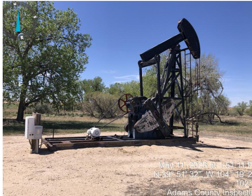
Photo # 3 Pump jack.
