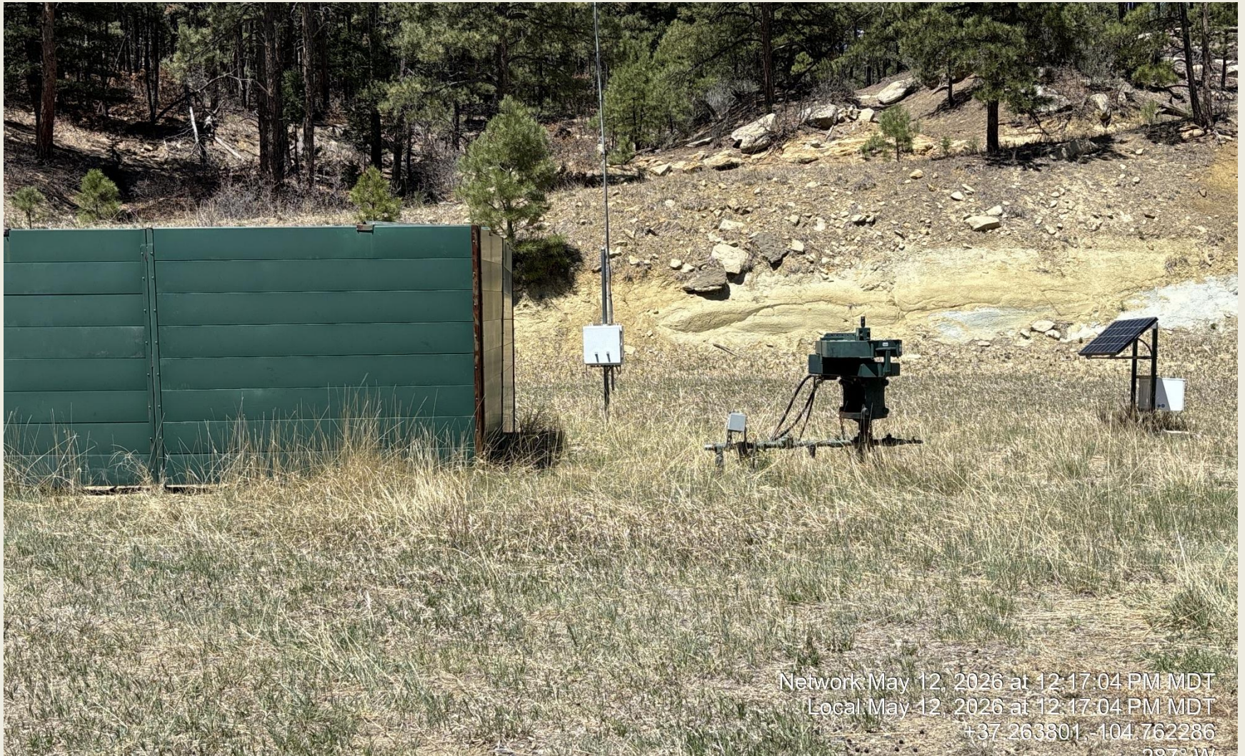
PHOTO 4: WELLHEAD AND EQUIPMENT. GRASS AROUND WELLHEAD, EQUIPMENT AND METERHOUSE IS NOT MAINTAINED. MAINTAIN GRASS/WEEDS AROUND ALL EQUIPMENT INCLUDING INSIDE SOUNDWALLS PER RULE 606. CA DATE 6/12/2026.
