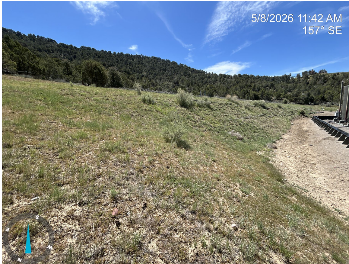
Photo 6: Photo showing eastern cut slopes are well vegetated. Overall, interim areas are progressing towards 1003 reclamation requirements.
