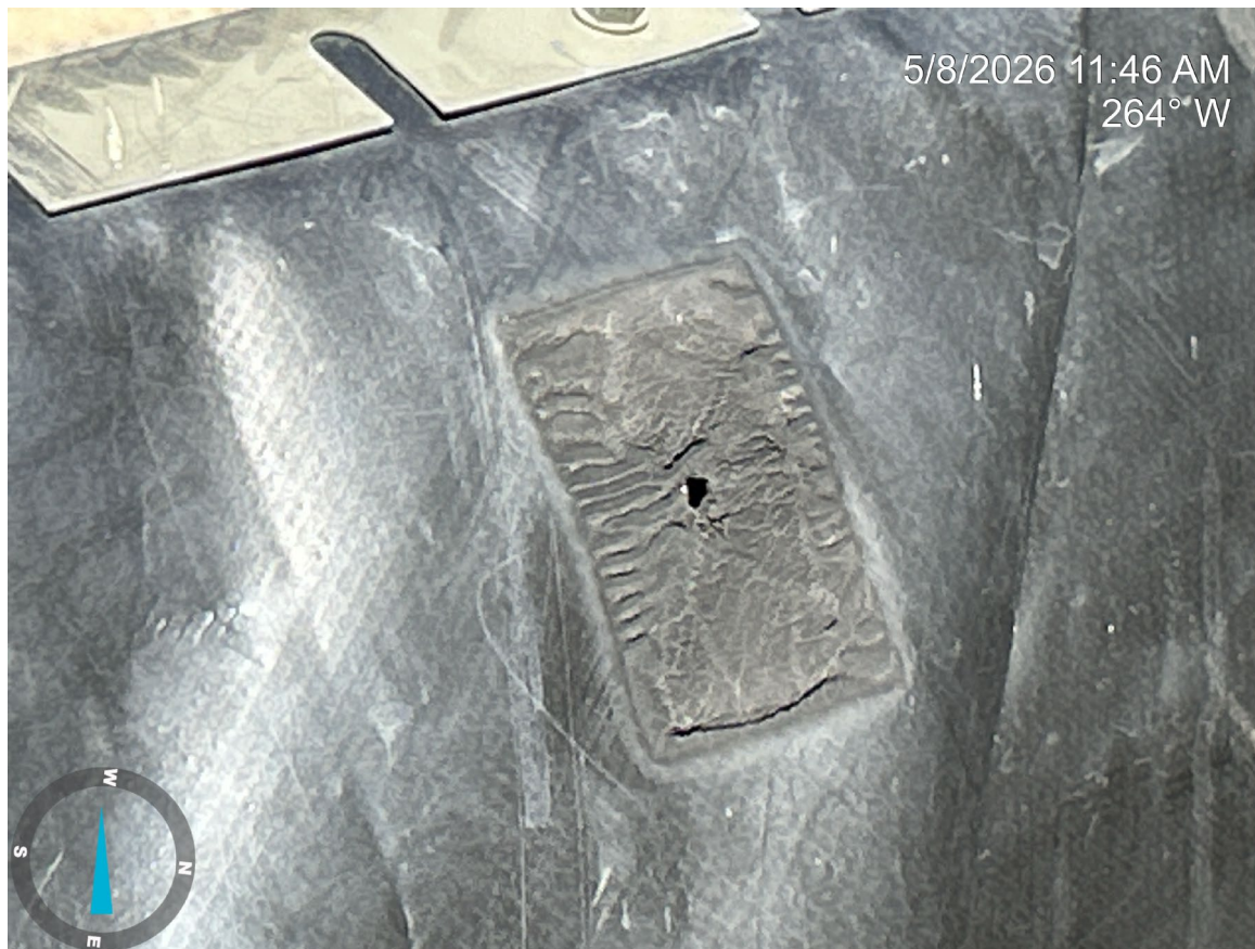
Photo 7: Photo showing a small hole is present in a patch at the tank's secondary containment black geotextile liner. Maintenance is required.
