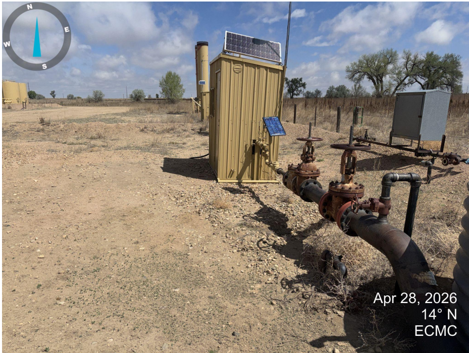
Photo 5. Looking north down the east side of the location.
