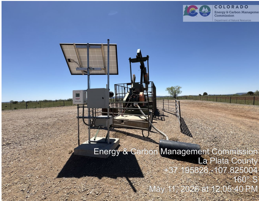
9. Solar telemetry for well controls. Muffler for prime mover on gravel.
