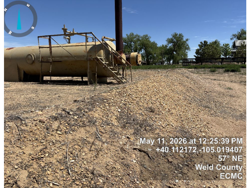
Photo 10: Berm repaired
