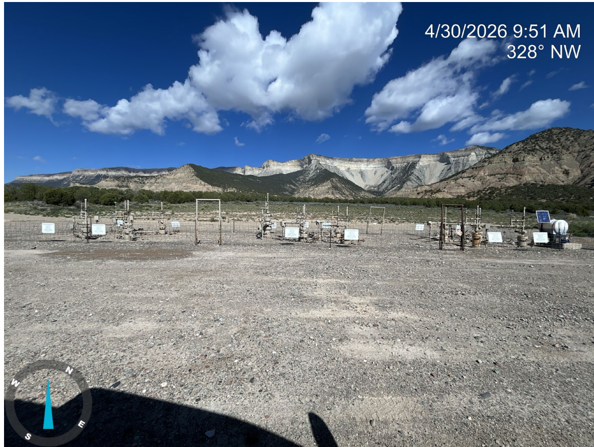
Photo 4: Photo showing an overview of the wellhead area.
