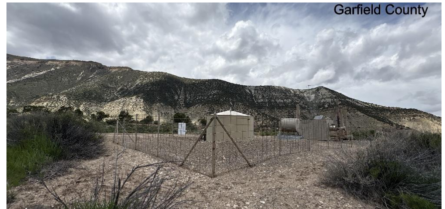
South East corner of location.
