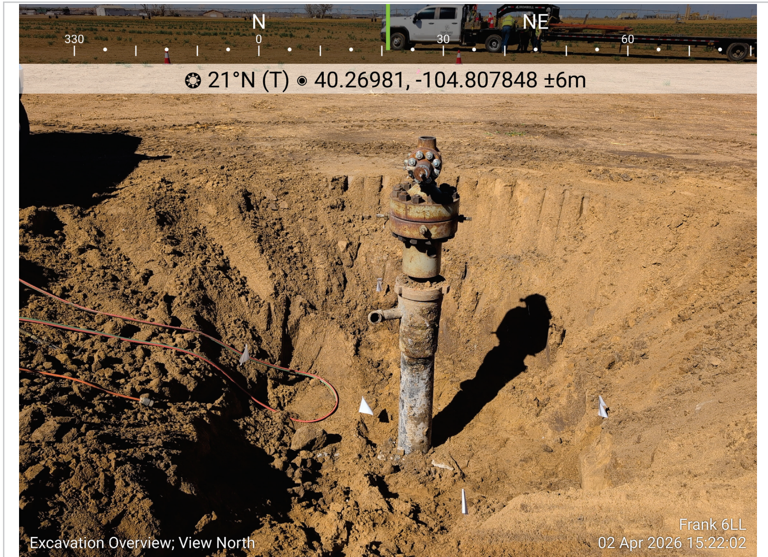
Excavation Overview: View North
