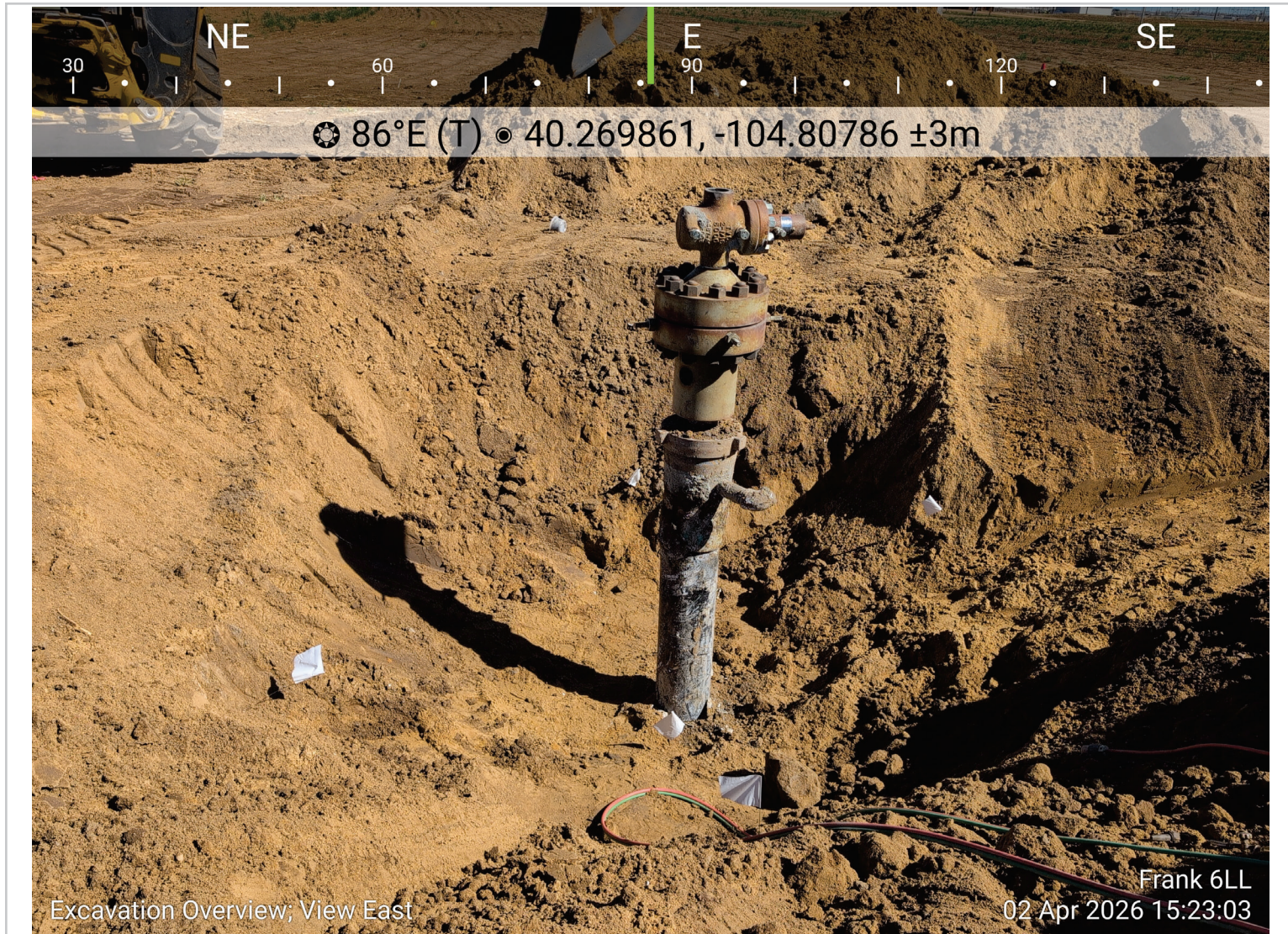
Excavation Overview: View East
