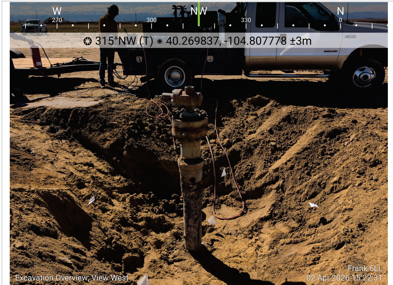
Excavation Overview: View Northwest
