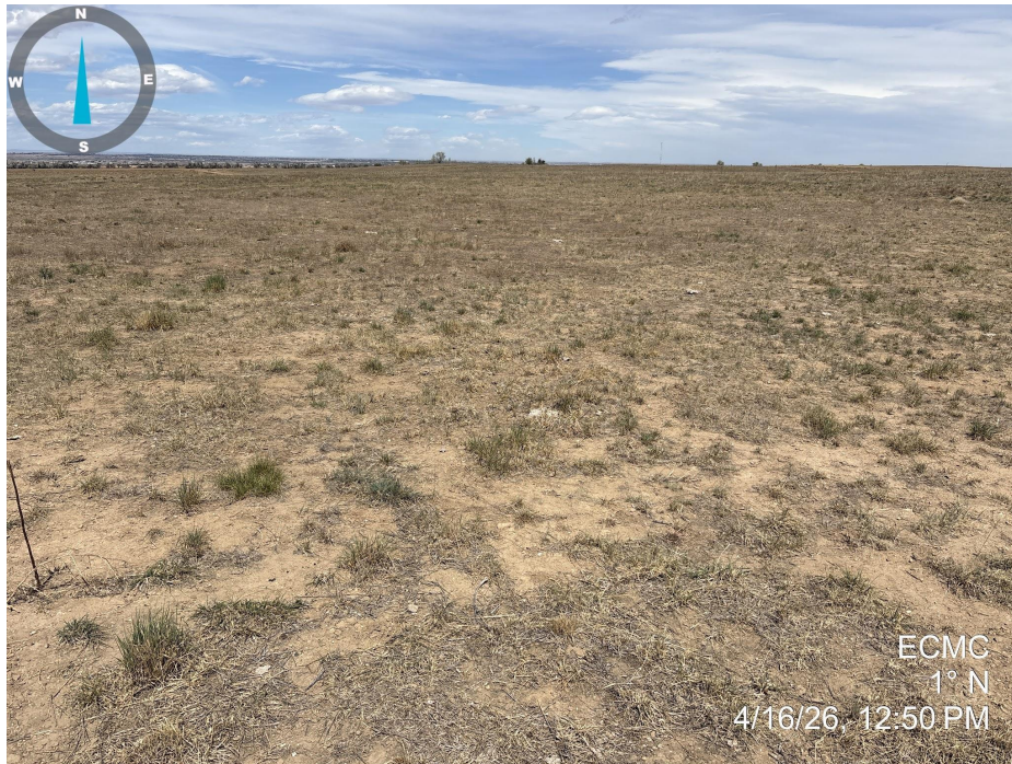
Photo 1. Photo taken of the multi-well location, facing north. Photo illustrates that final reclamation activities appear to have taken place, but vegetation establishment does not meet Rule 1004 standards.
