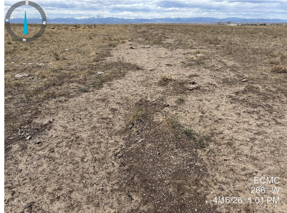
Photo 6. Photo taken of the access road to the well location, facing west, towards the location. Photo illustrates that final reclamation activities appear to have taken place along the access road, but vegetation has not established to Rule 1004 standards and bare ground and mulch were observed.
