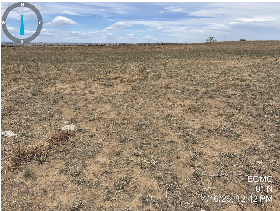
Photo 1. Photo taken of the well location, facing north. Photo illustrates that final reclamation activities appear to have taken place, but vegetation establishment does not meet Rule 1004 standards. Weedy annual vegetation including russian thistle ( Salsola tragus ) and cheatgrass ( Bromus tectorum ) were observed at the location.
