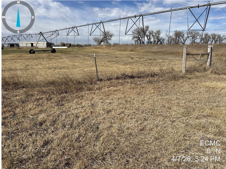
Photo 1. Photo taken of the well location, facing north. Photo illustrates that final reclamation activities have taken place and vegetation appears to have established to Rule 1004 standards. However, subsidence was observed at the well location.
