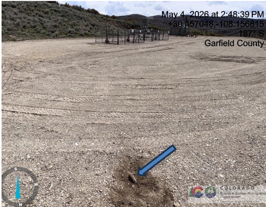
Photo # 5431 Same unmarked deadman
