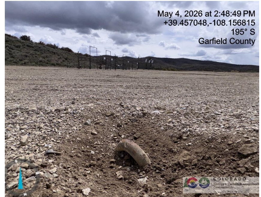
Photo # 5432 Same unmarked deadman
